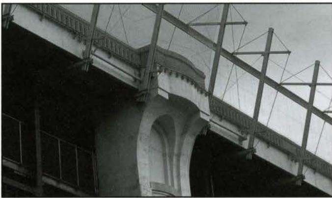
Fig. 9: Typical lookout at top of bridge pier.
