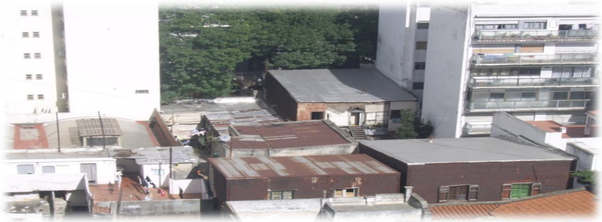
Picture 2.4: Shacks and improvised houses in the heart of La Boca.
