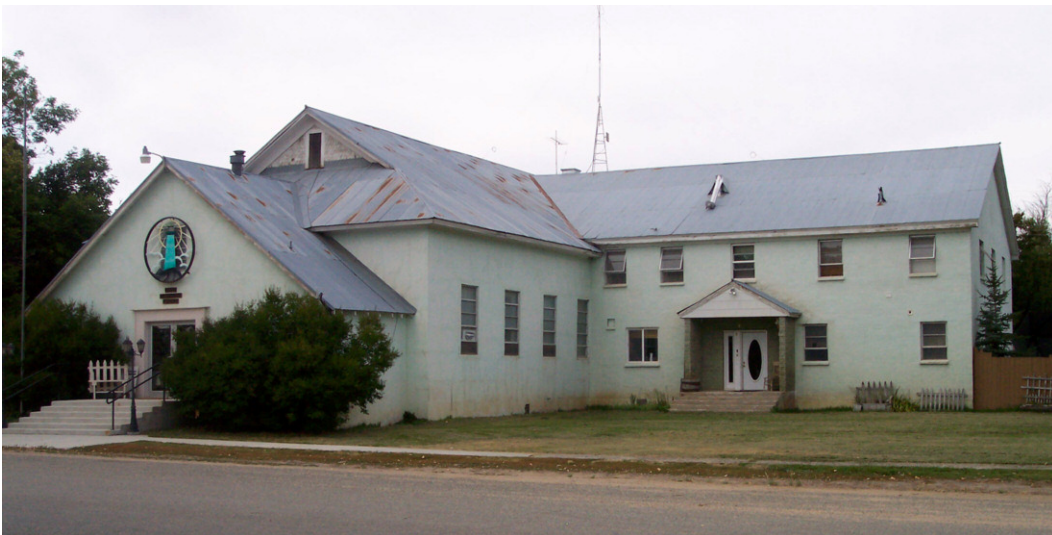
On the right is the extension added after it's moved to Fairfield with extra classrooms, Relief Society room, kitchen and rest rooms. Also the little front section (on left) with entry way was not part of the original building.
