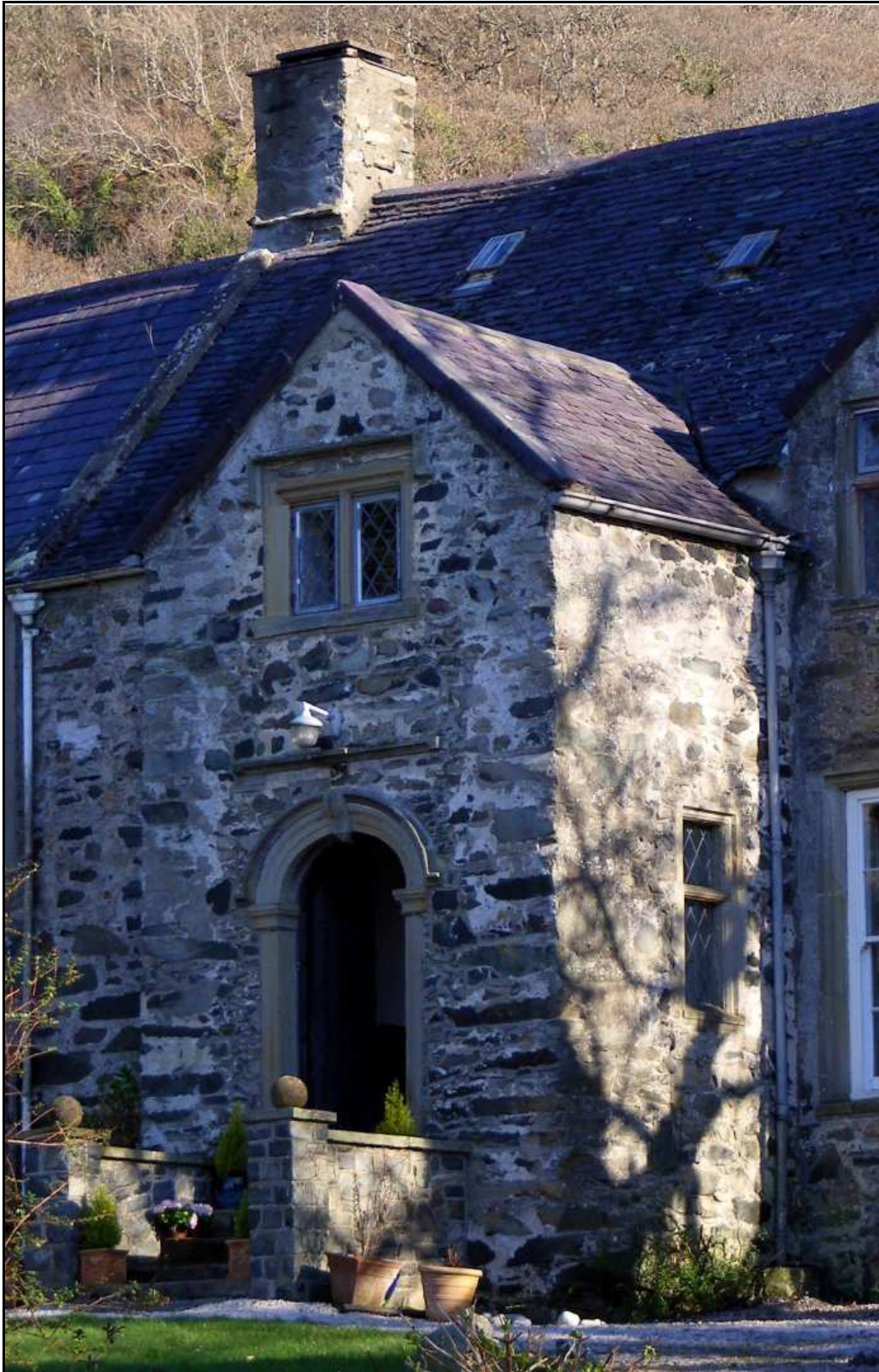
Figure 60 , The porch (P) showing the different roof lines between this building and the main house (H).
