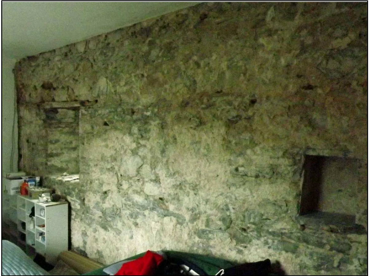
Figure 52 , The interior western wall of the first floor of the south range (S) showing the stone cupboard with window embrasure beyond.
