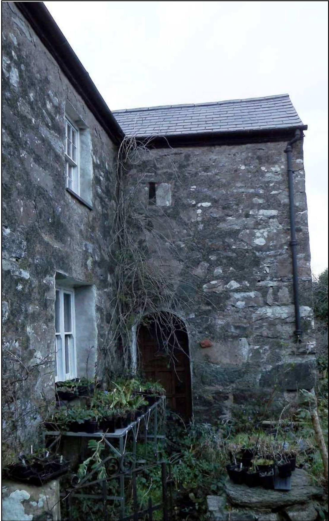
Figure 61 , The porch at Penhyddryn near Nefyn.
