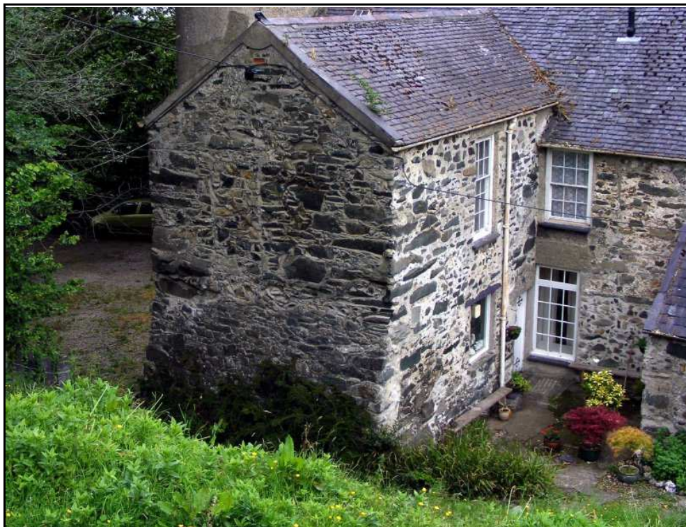
Figure 45 , The south wall of the south range (S) from the hillside. Notice the ghost of the blocked south door into the possible first floor garderobe.
