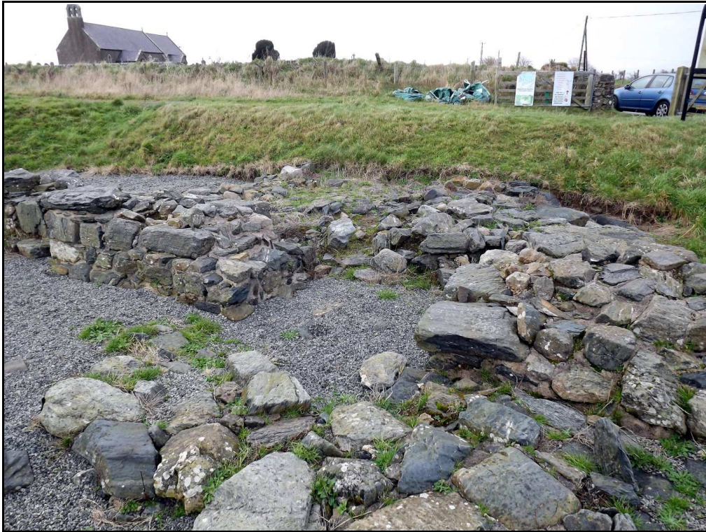
Figure 79 , The rear of the east gateway at Rhosyr from the building D. Note the walling filling the entrance and the nearby church of St Peter in the background.
