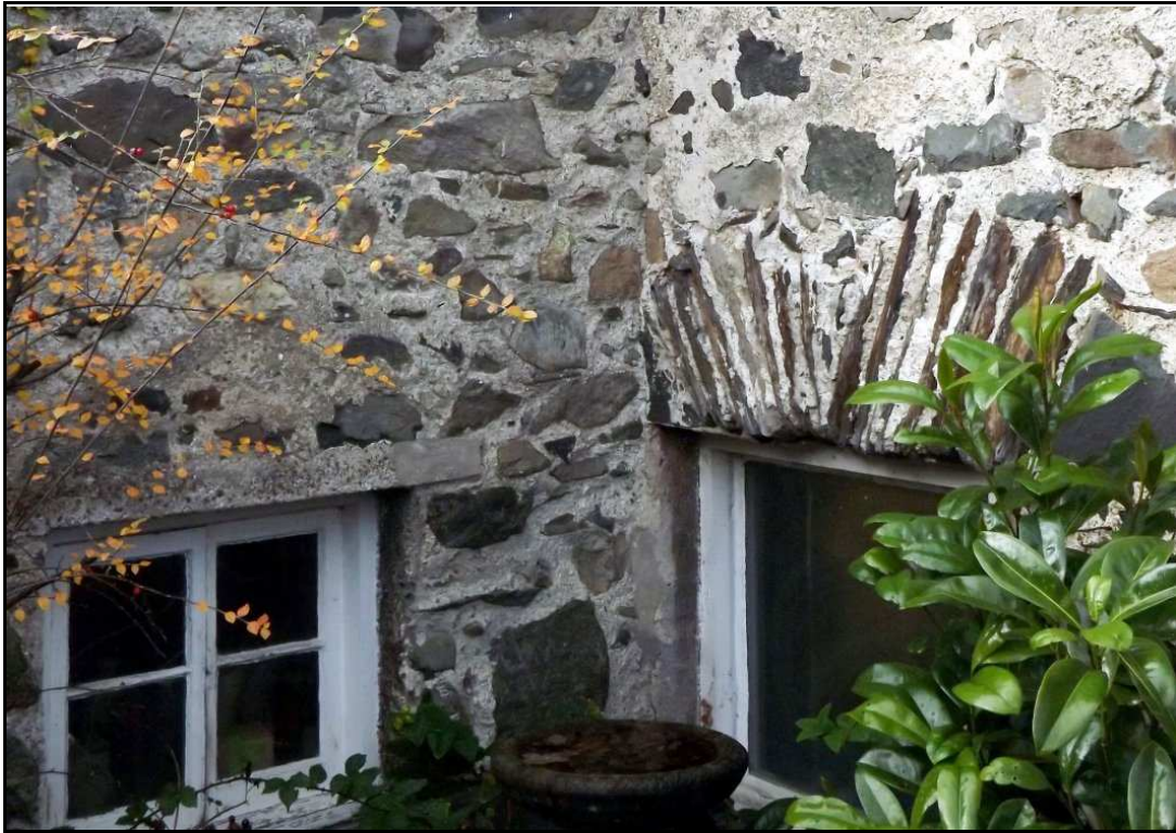
Figure 27 , The south-eastern voussoir in the east range (E) next to the more modern tool shed.
