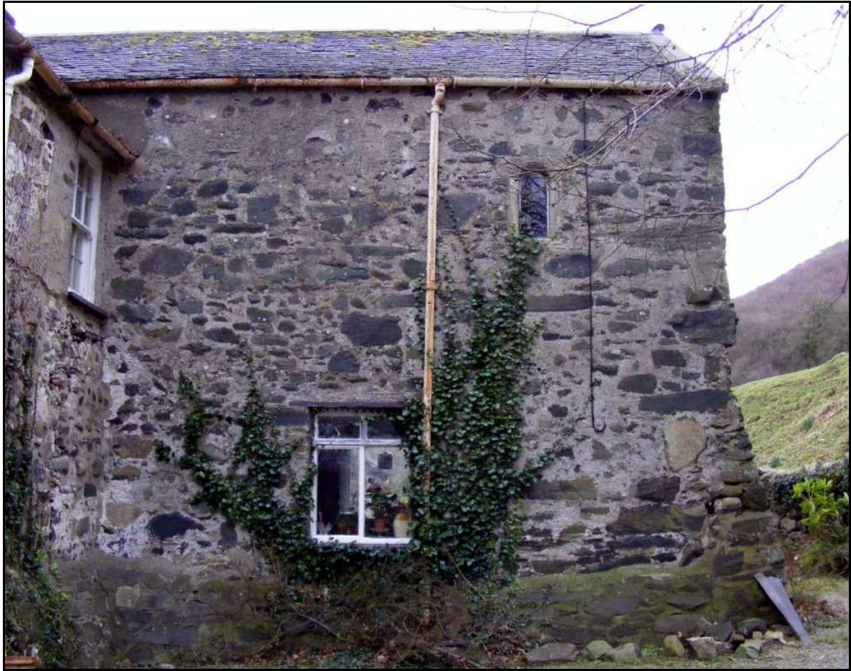
Figure 48 , The south range (S) from the west.
