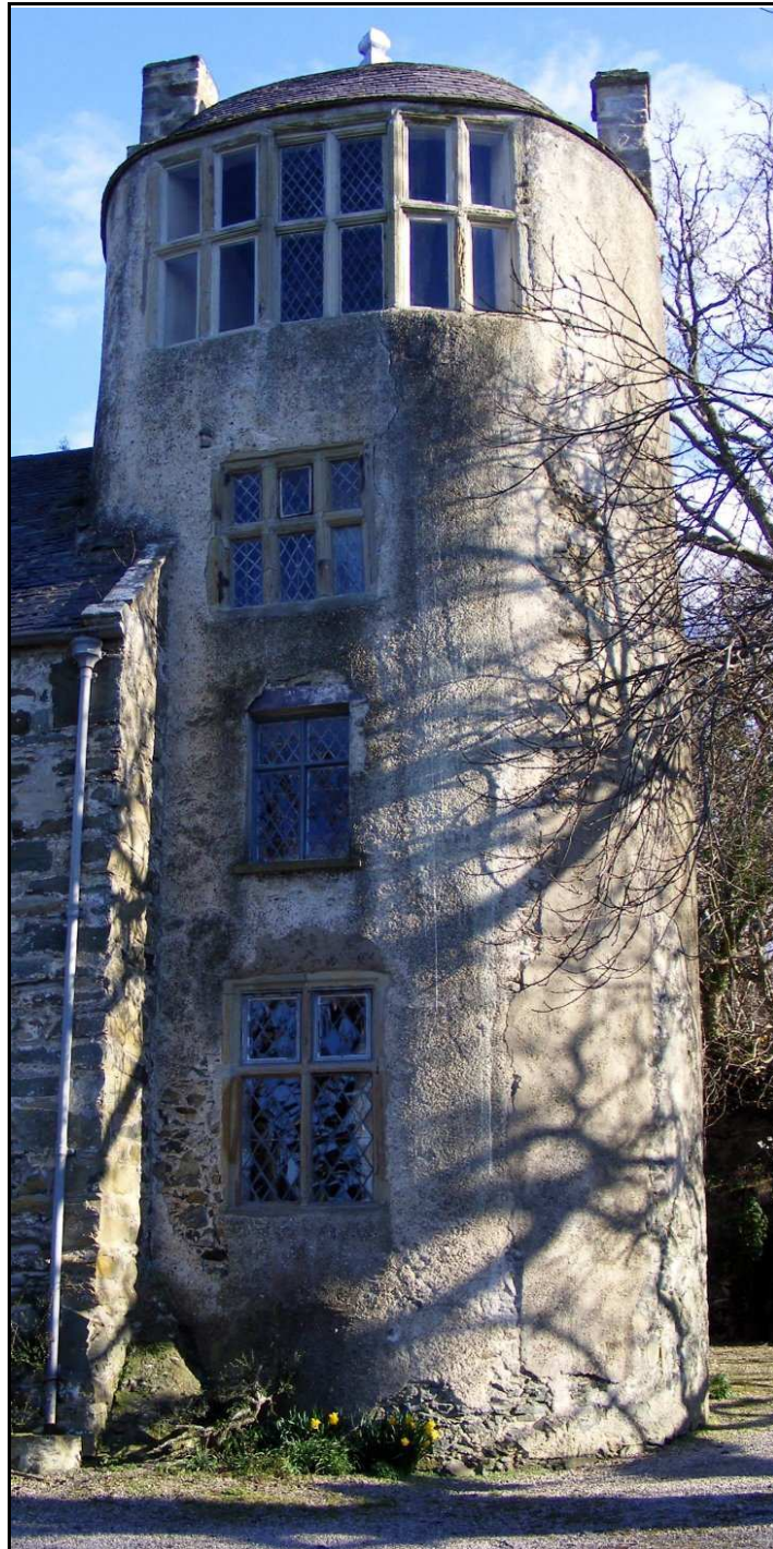
Figure 63 , Llywelyn's tower (T) from the north.
