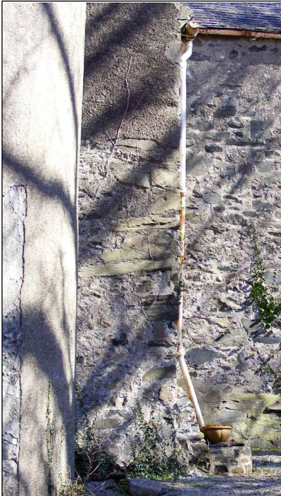
Figure 38 , The south-western corner of the house (H) where an apparent doorway has been walled up. Notice the later still sloping plinth under the downpipe next to the drain. The tower (T) is to the left and the south range (S) to the right. The lintel of the blocked doorway is the green schist-like stone that stretches right across the wall.
