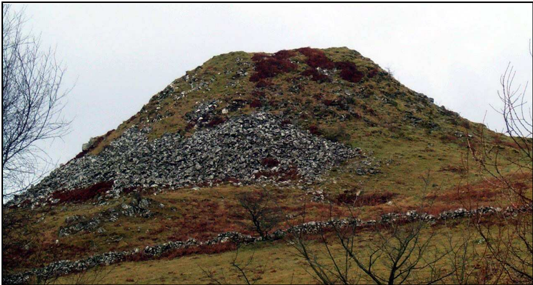
Figure 28 , The ‘motte’ at Castell Prysor. This is not in fact a motte, but the collapsed remnants of a tower which points out dramatically the problems of not remortaring on a regular basis when using uncoursed masonry.
