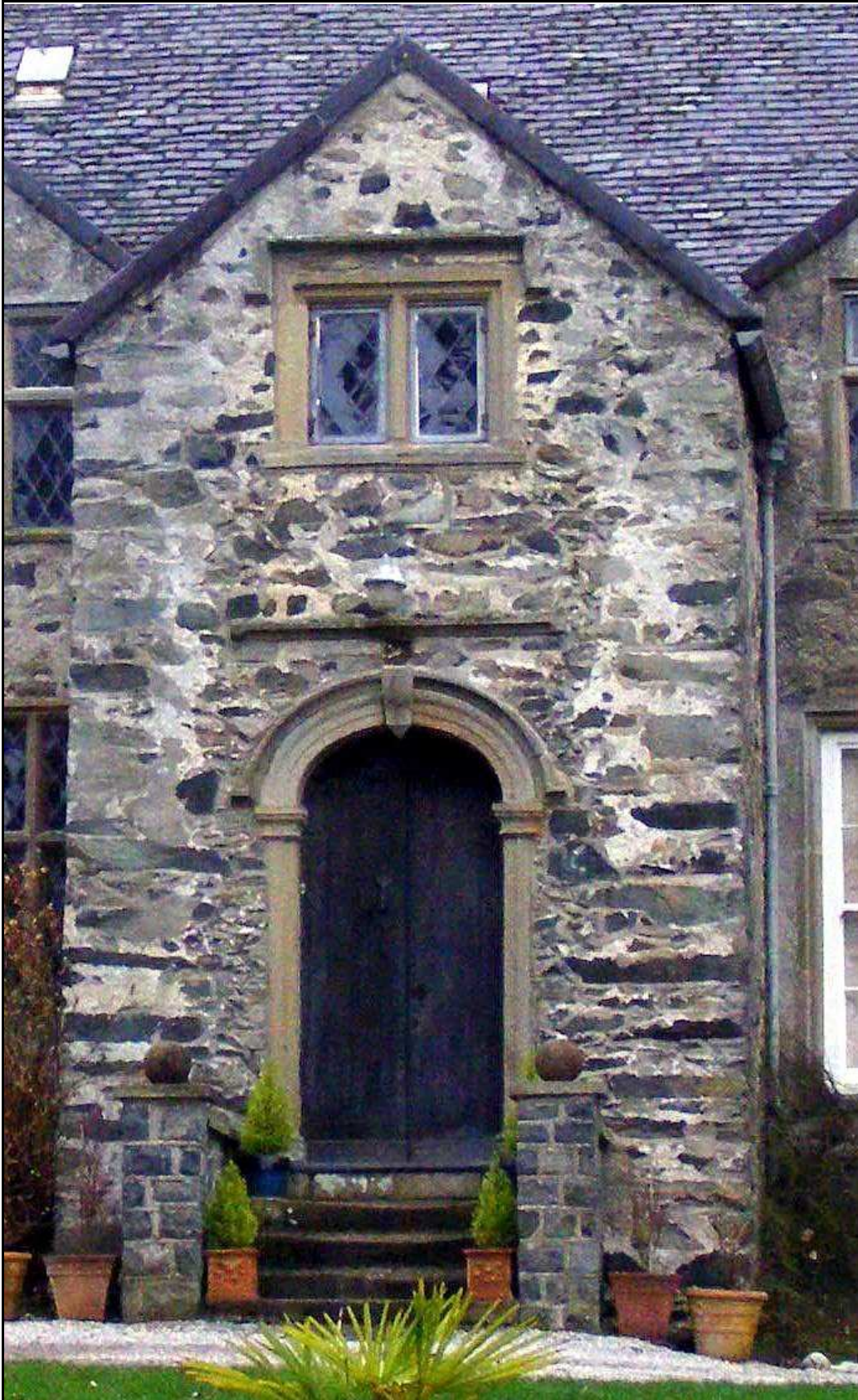
Figure 56 , The entrance to the porch (P). Notice the change in masonry style between the phase 2 quoins and the tertiary insertion of the doorway and its string course above. The masonry above the window looks similar to that in the phase 1 side walls.
