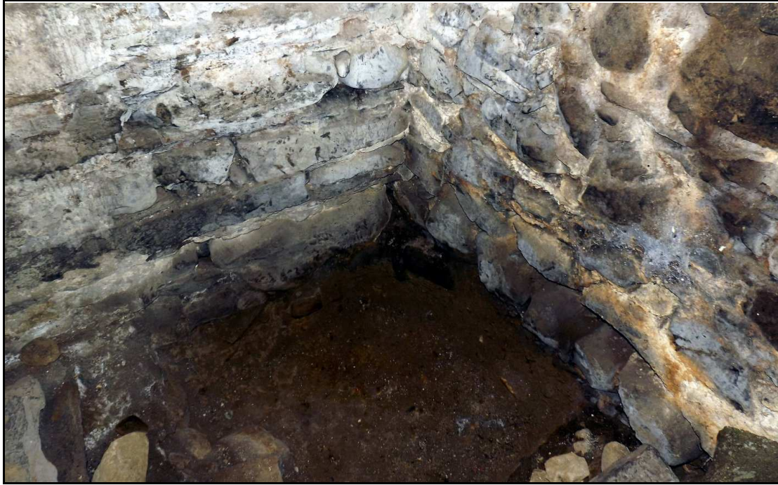
Figure 34 , The north-east corner of the fireplace showing the replacement east wall of the east range (E) resting on a row of water washed sandstone boulders to the bottom right. The chimney north wall to the left can be seen to make butt joint with the older east wall.
