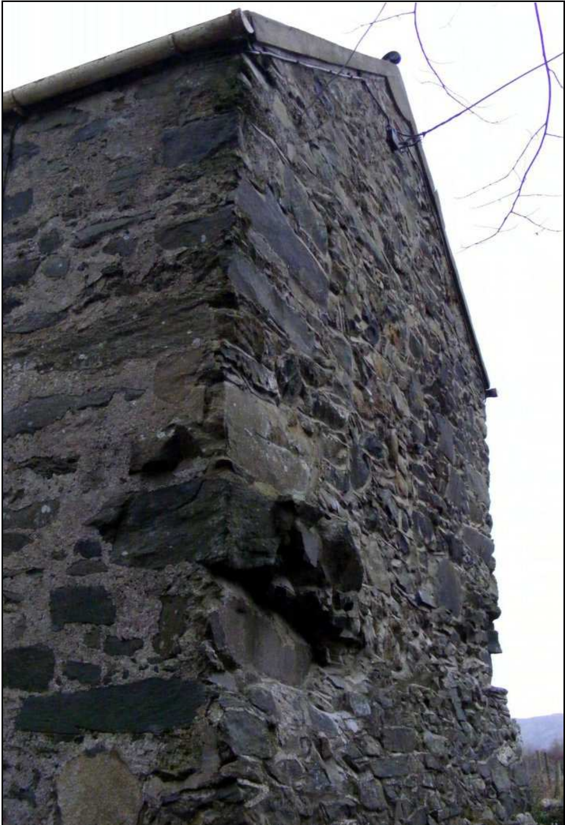
Figure 43 , The southern end of the south range (S), showing the line of the projecting first floor level and the large, replaced corner quoins above. The top of the added sloping plinth can be made out at the bottom of the picture.
