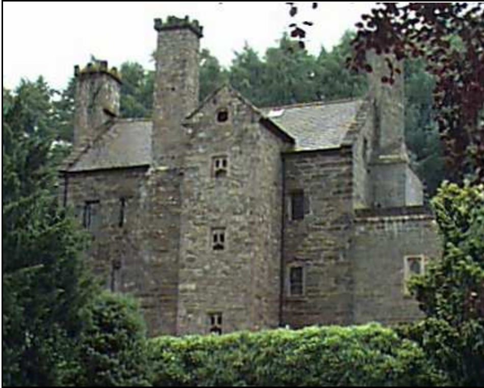
Figure 85 , The early sixteenth century block at Gwydir from the north. Notice the 'mid sixteenth century' stair turret in the foreground which bares comparison to the porch (P) as it appeared in the Colt Hoare picture (Fig.22).
