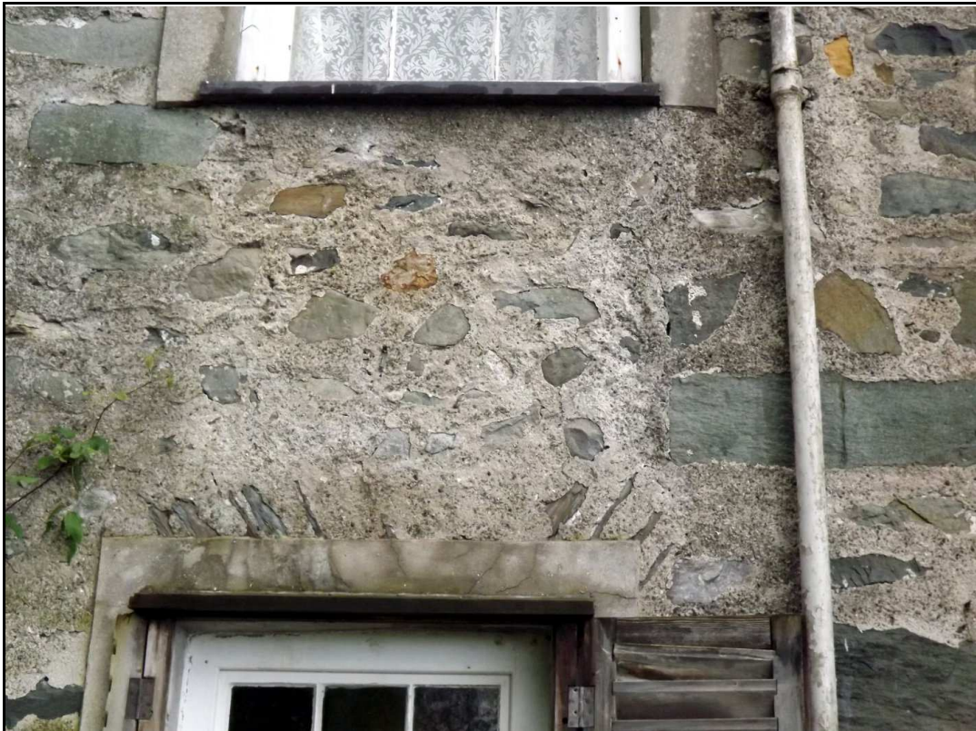
Figure 21 , The clear junction between the irregular rubble of the east range (E) to the left, and the more coursed masonry of the house (H) to the right, occurring between the drainpipe and the window edges.
