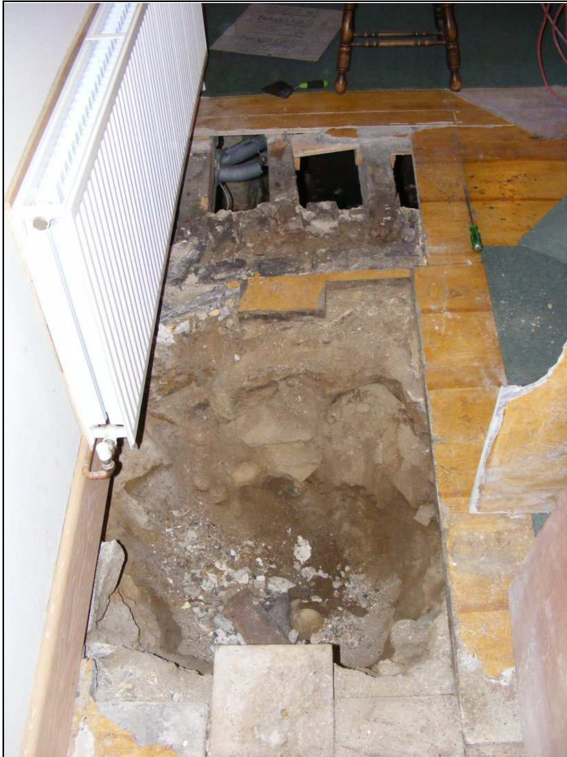
Figure 9 , The shallow excavation into the rubble fill in the south-western portion of the basement (B) from the southern range (S) door. The retaining wall and the north-western cellar can be seen under the joists in the background.
