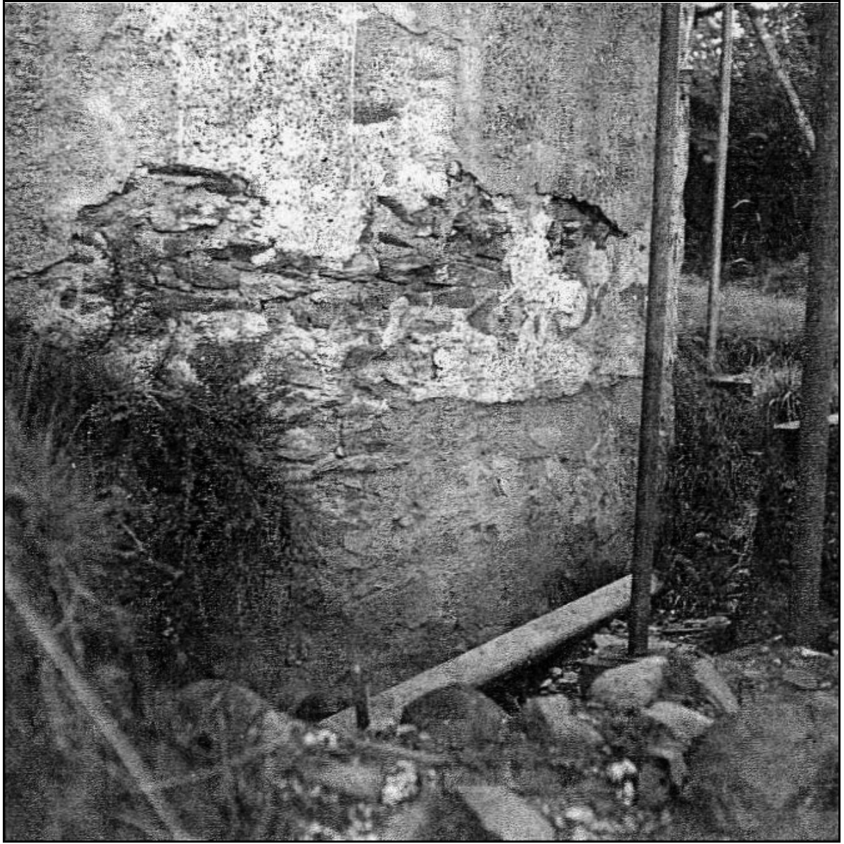
Figure 64 , A buried portion of the tower (T) when uncovered during the excavations of 1993.
