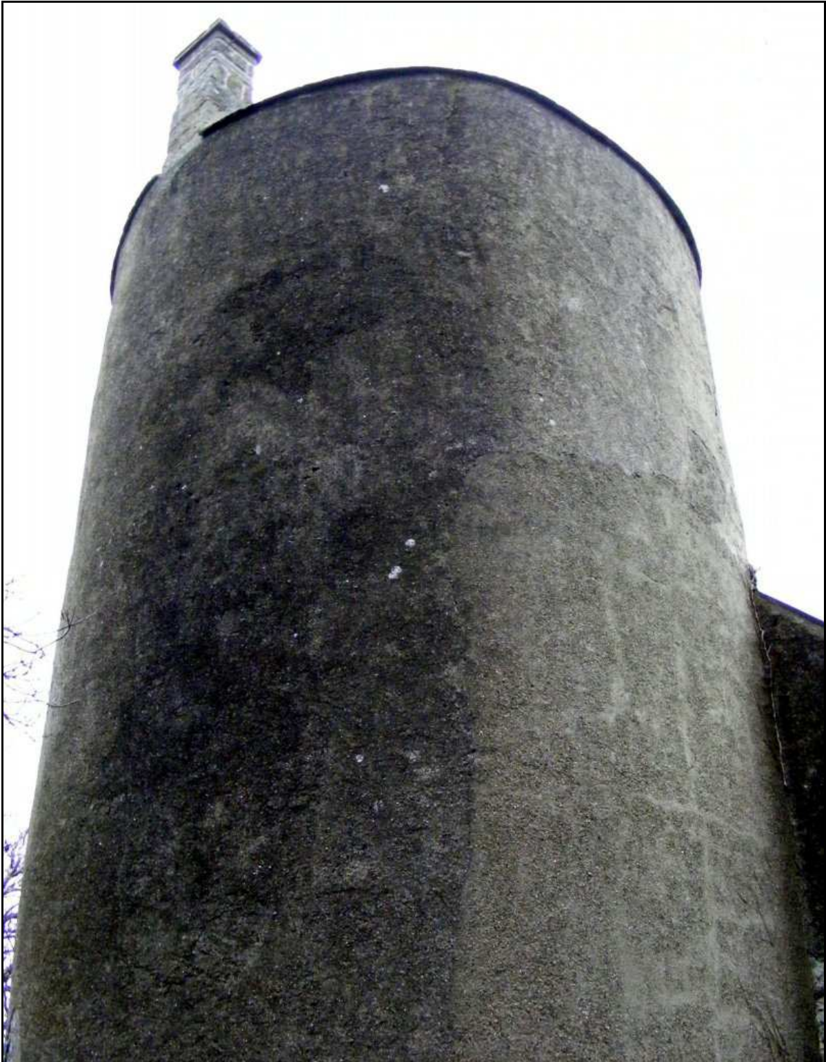
Figure 67 , The western face of the tower (T) showing a rectangular depression on the third floor. An original window here to overlook the town is a distinct possibility.
