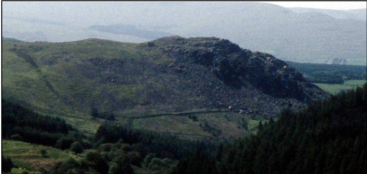
Figure 29 , Castell Carndochan from the east. Again see what remains of the castle stone strewn over the hillside after a catastrophic failure of the walls once the mortar rotted away.
