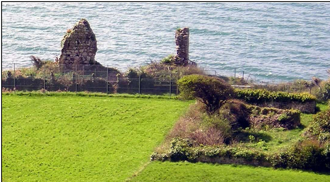
Figure 30 , The collapsed remnants of Gogarth hall to the right. The lack of rubble on the site could either be due to the 1950's excavations or the reuse of materials from the collapsing walls.
