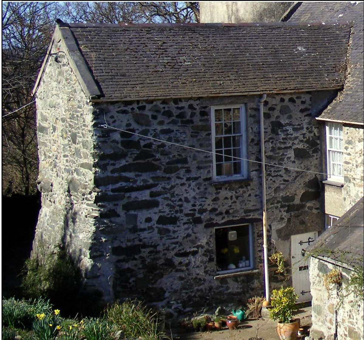
Figure 42 , The south range (S) from the east.
