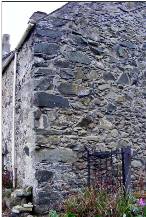
Figure 32 , The southern corner of the east wall of the eastern range (E). Notice the large quoin stones and the different masonry style of the east wall.
