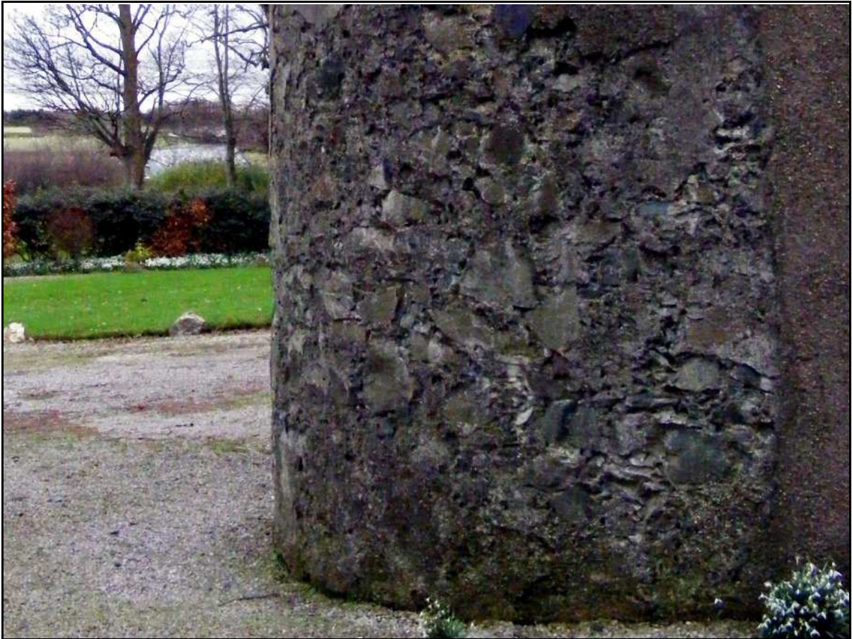
Figure 68 , The base of the tower (T) showing the distinctively irregular make up of the masonry.
