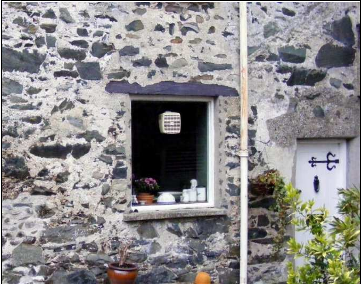
Figure 46 , The eastern window of the south range (S) showing its slate lintel and much rubble packing underneath and on either side which consists of smaller pieces of stone than the rest of the wall. The modern door to the north has a concrete lintel.
