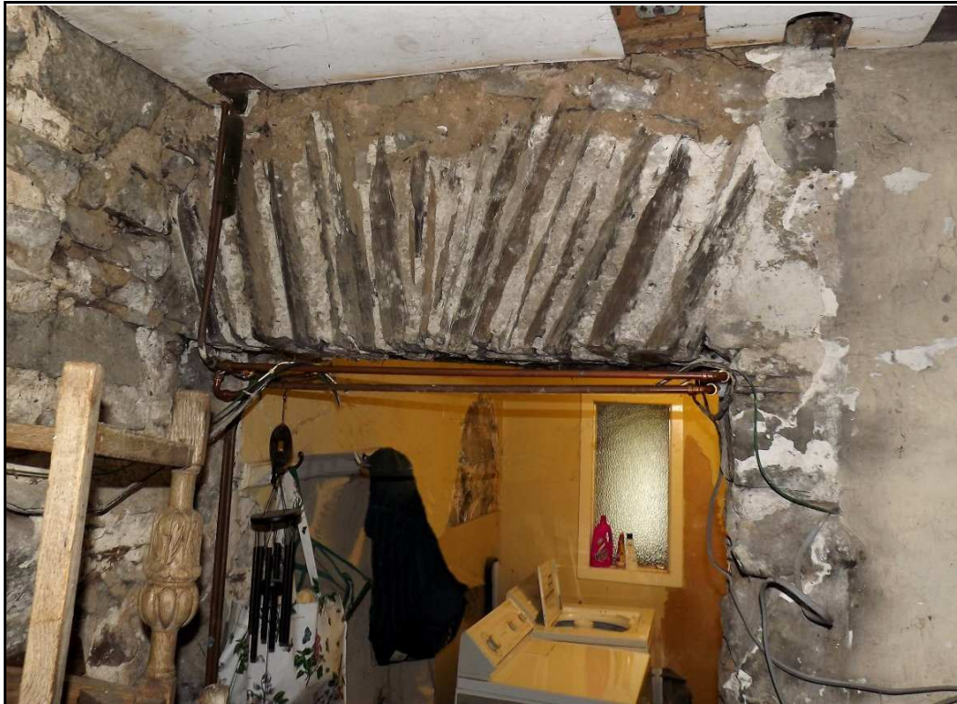
Figure 19 , The voussoir in the external south wall of the east range (E) from the tool shed. Notice how it penetrates the wall of the house (H) to the upper left.
