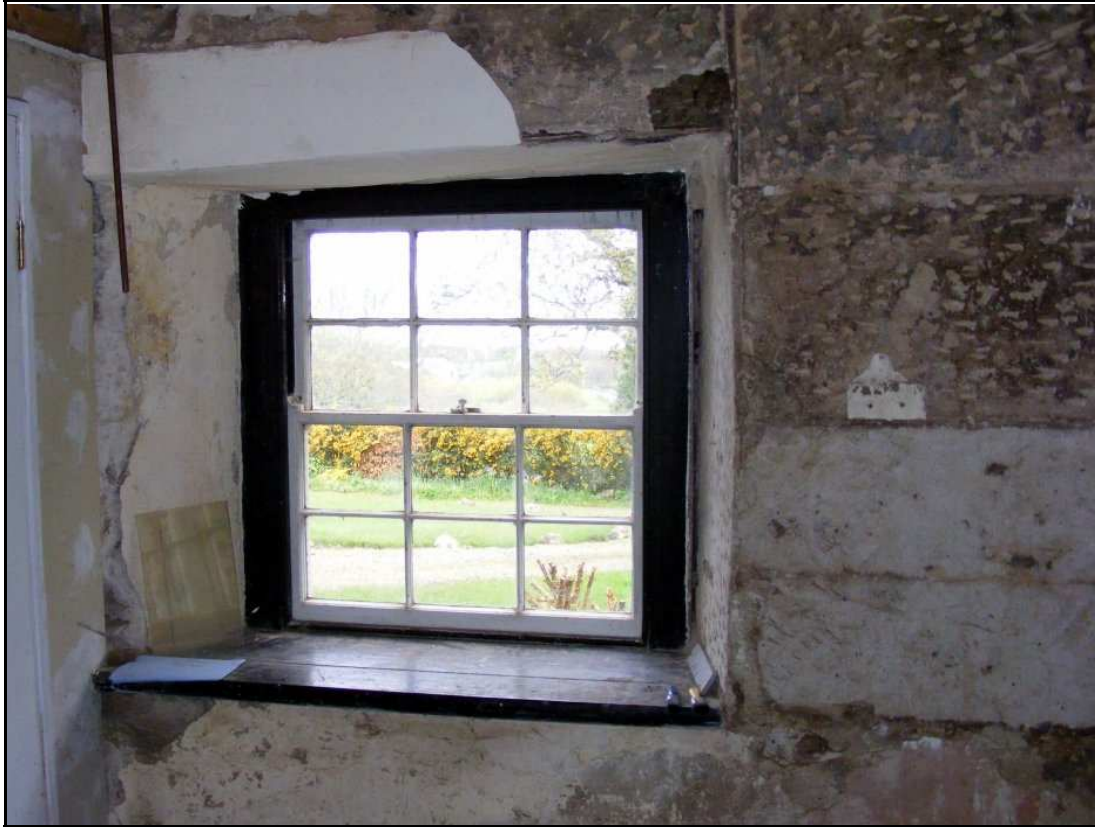
Figure 25, The north-eastern window embrasure of the east range (E).
