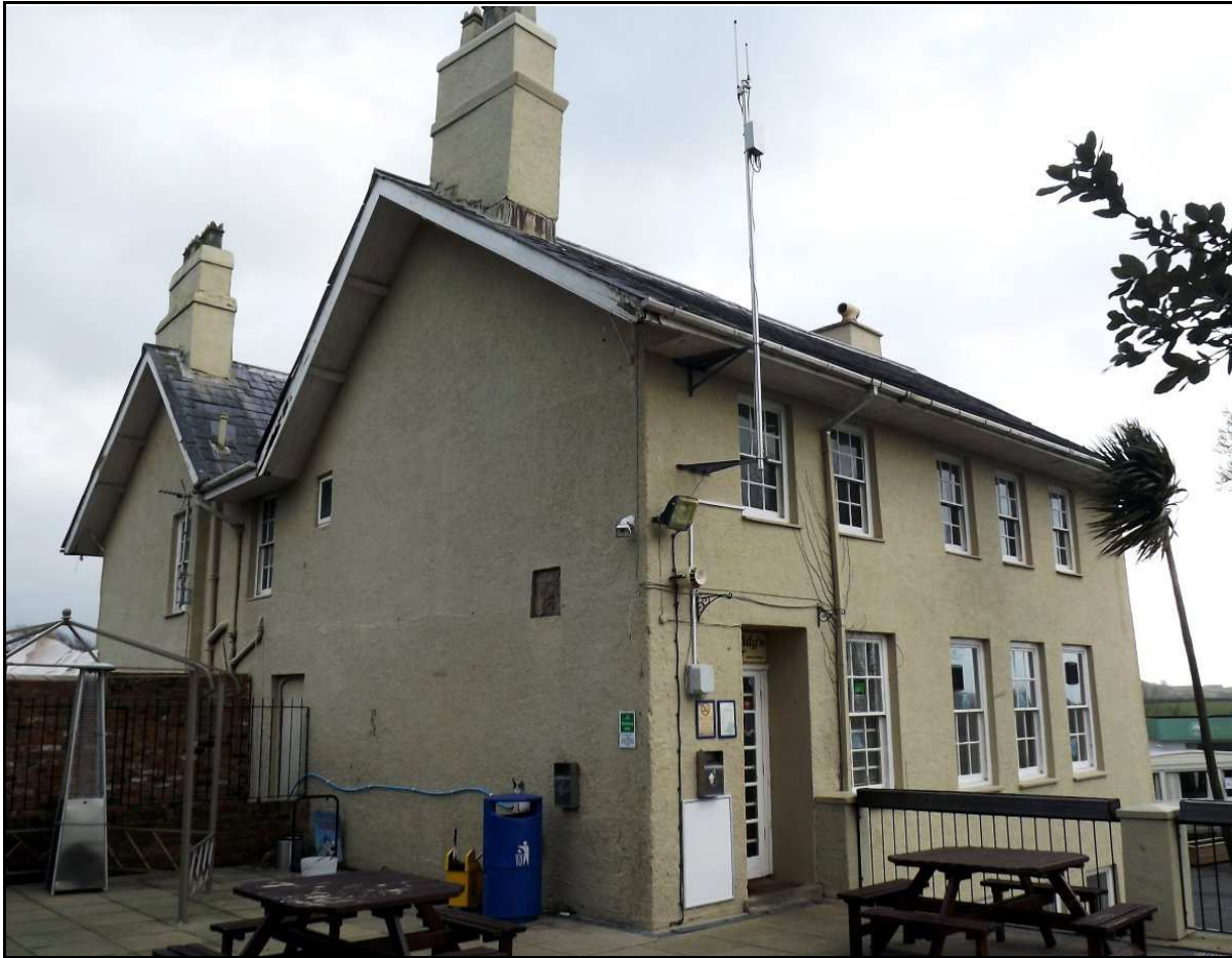
Figure 88 , Coed Helen from the south showing the twin gabled blocks of the probably original build. The ground floor is currently buried under the patio in the foreground on this front.
