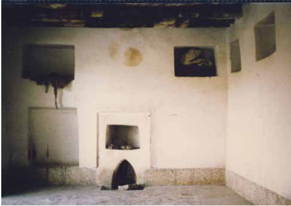
Fig. 8. The ôjâgh in the takya .
