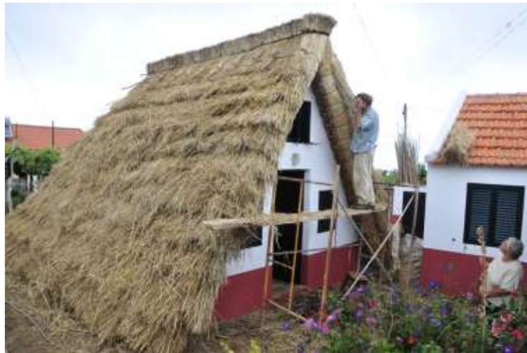
Figure 13. Roof straw thatching in a Santana typical house
