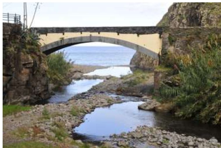
Figure 40. Bridge over Ribeira de São Jorge stream
