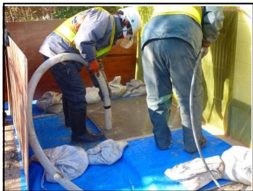
High pressure water cleaning of paved road
