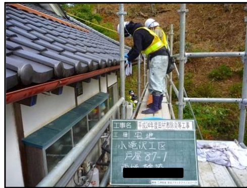
Wiping off a gutter
