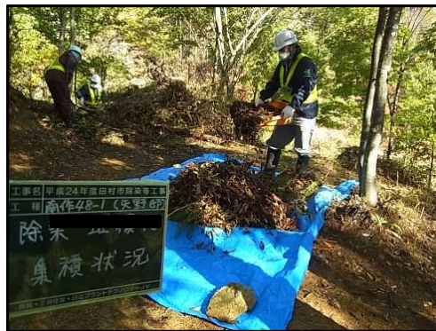
Mowing and removal of sludge
