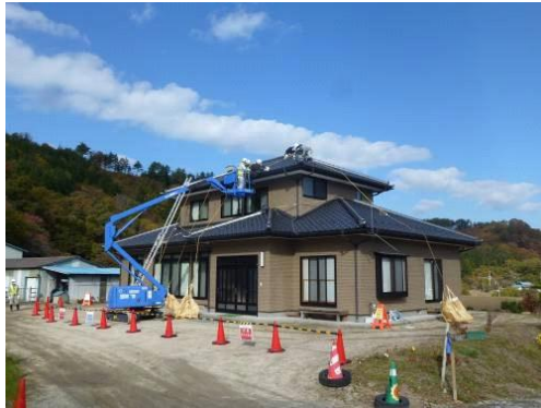
Wiping off rooftop and walls
