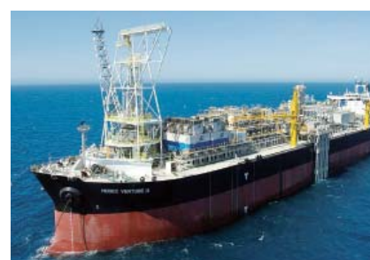
Floating storage and offloading unit
