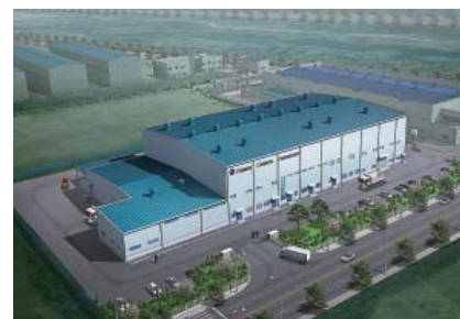
Plant for production of lithium-ion battery anodes under construction in South Korea
