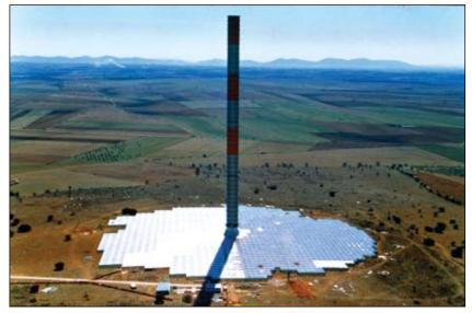
Fig. 3: The prototype solar chimney.
