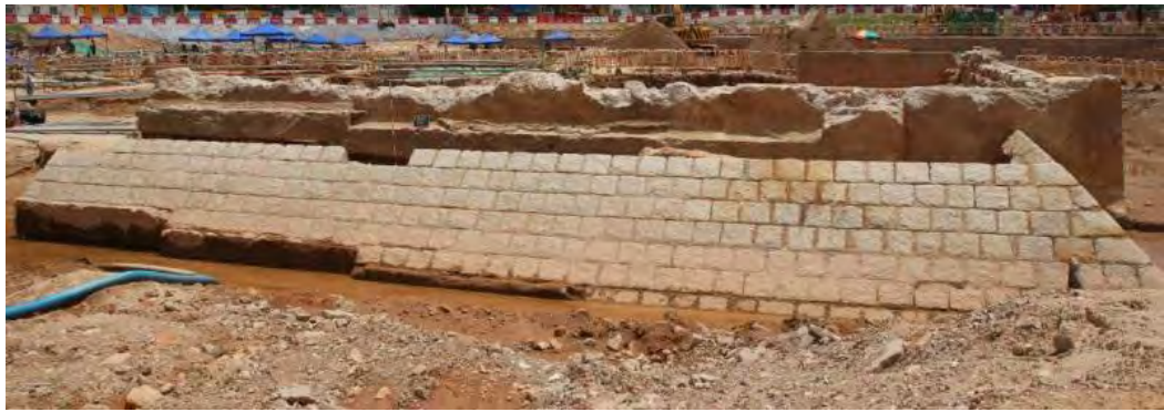
Figure B1c SW facing wall of SQ5
