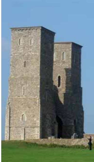
View of Reculver Towers from south - extraordinary investment in tower construction for a parish church
