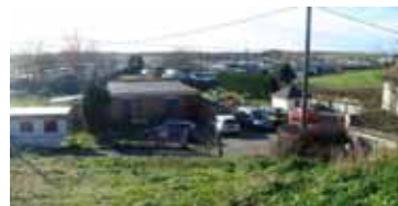
Poor frontage to the King Ethelbert Inn land
