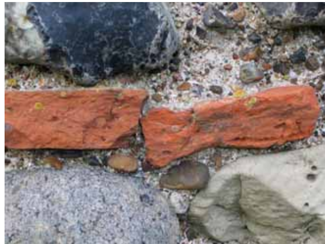
Detail of Roman Wall - clear evidence of construction method and materials
