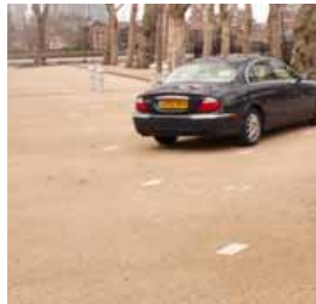
Bound gravel to main car park
