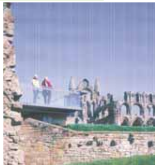
New structures to aid safe access
