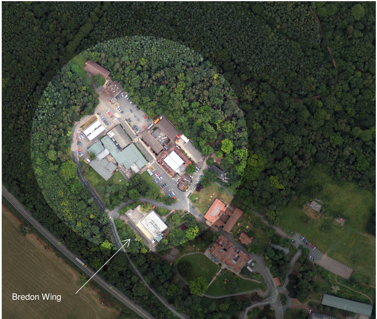
Aerial view of Wood Norton Campus
