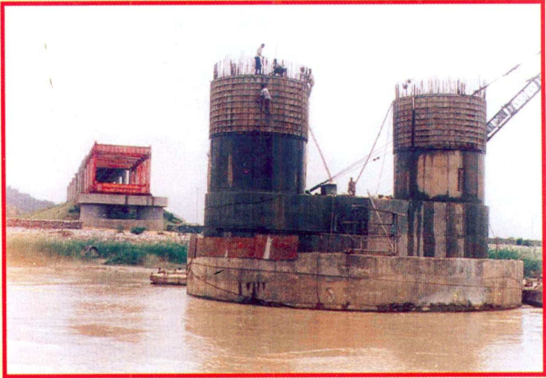
Construction of twin pier pedestal is going on
