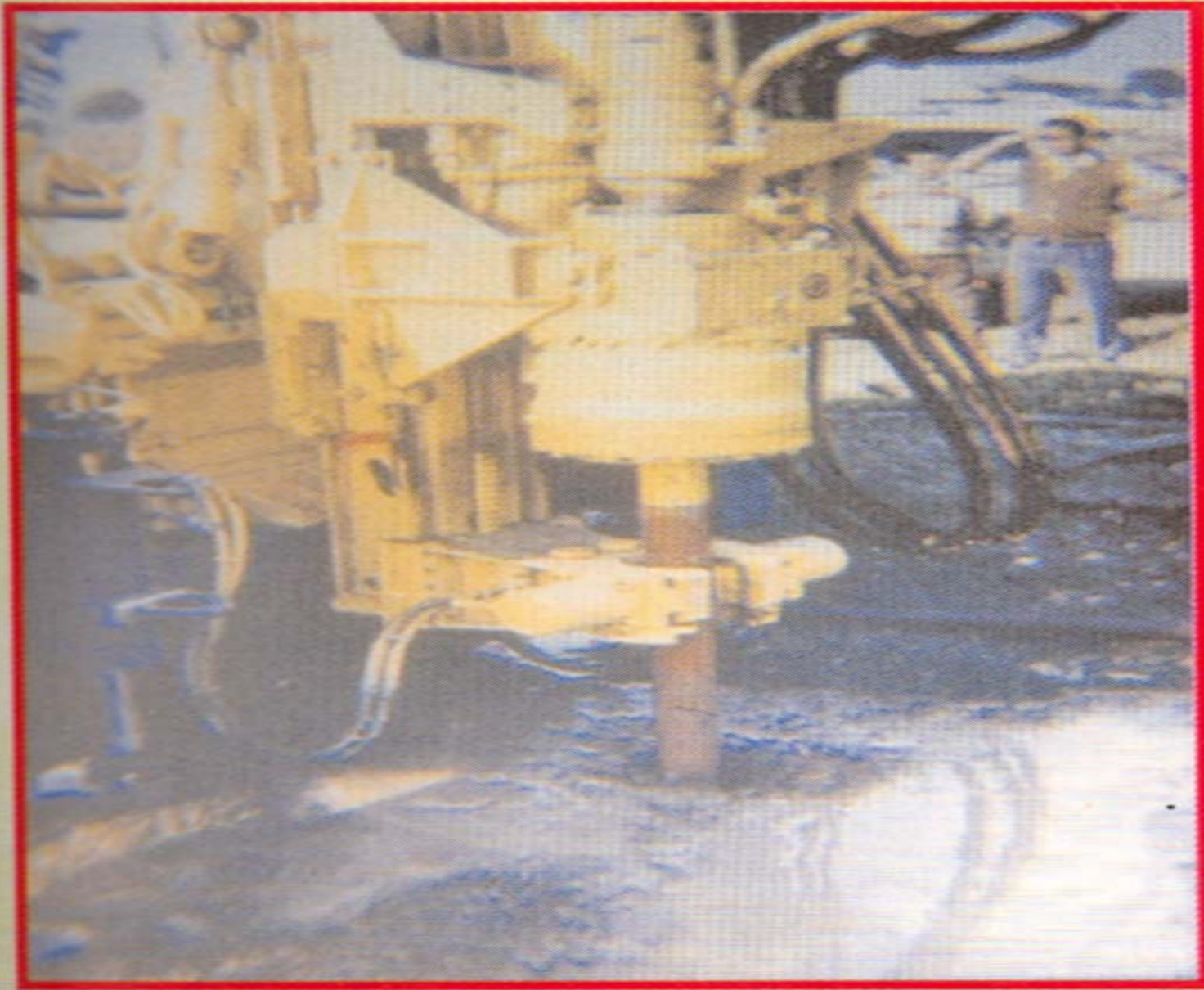
Jet grouting equipment used in construction of special Foundation ( Pier-17 & 18 )
