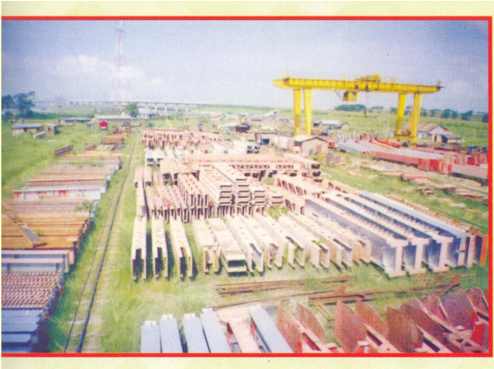
Fabrication and assembling yard
