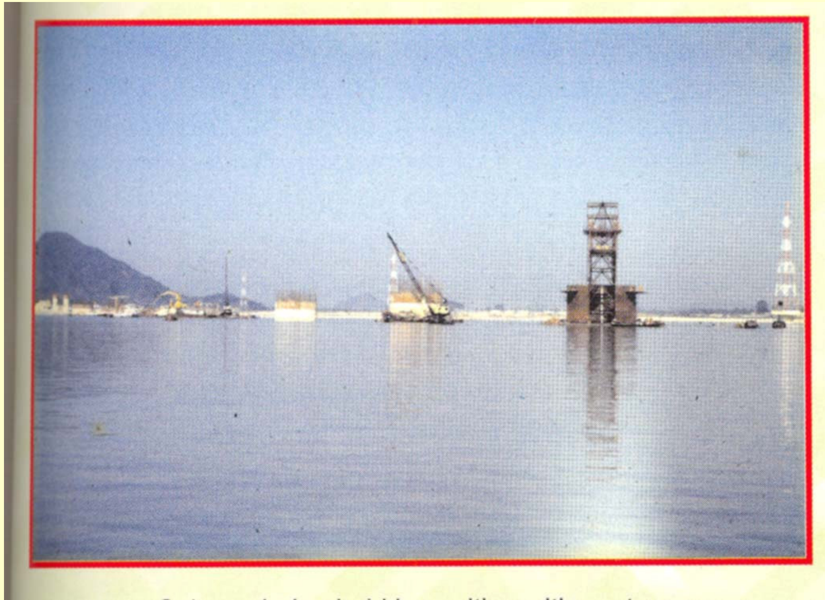
Caisson being held in position with gantry
