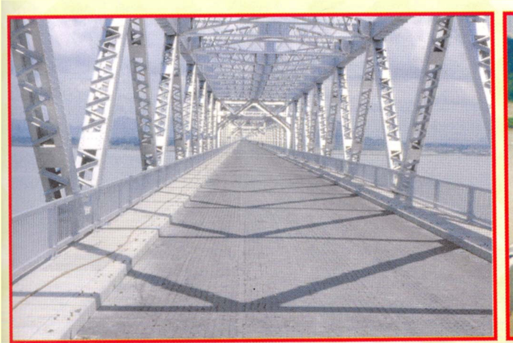
Completed road deck
