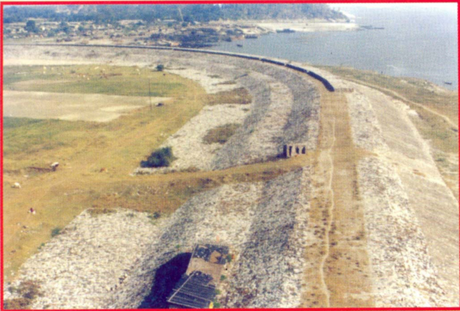
Completed portion of north Guide bund
