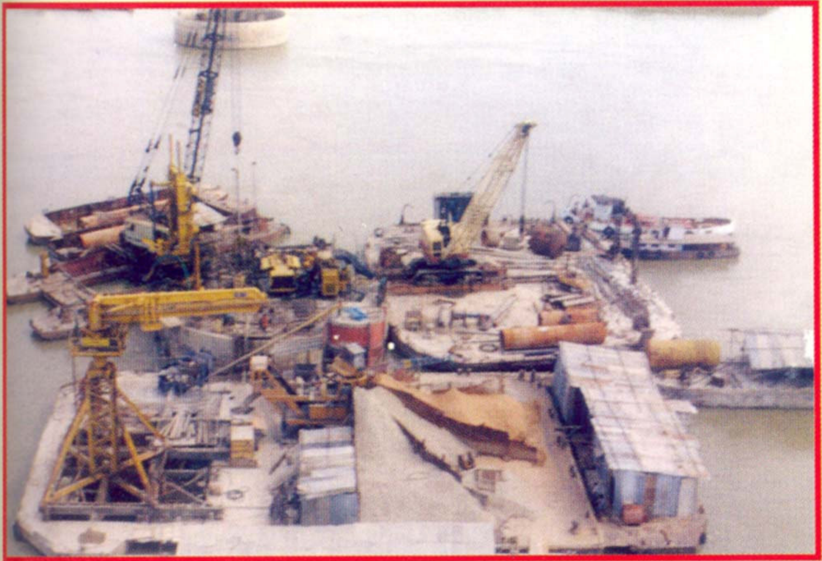
Barges carrying jet grouting equipment, rock drilling machine
