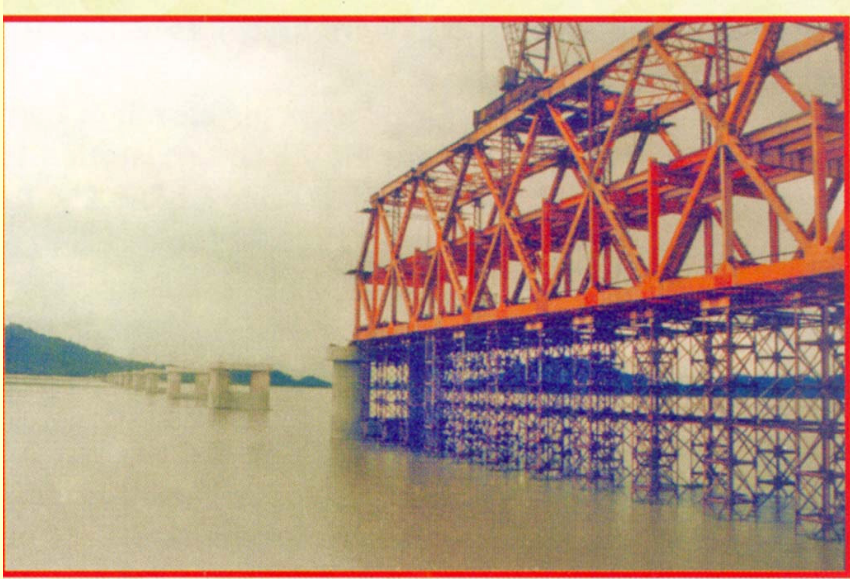
1 st anchor span at JPZ end erected on trestle
