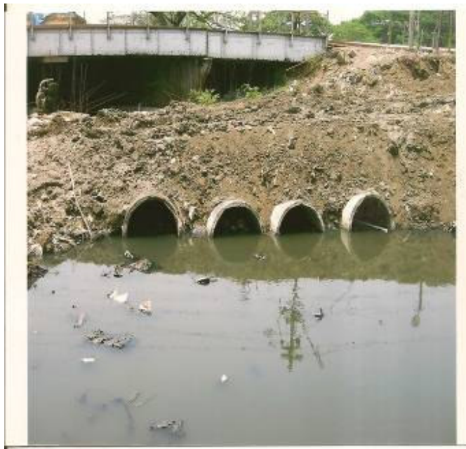
Photograph showing Approach Road
