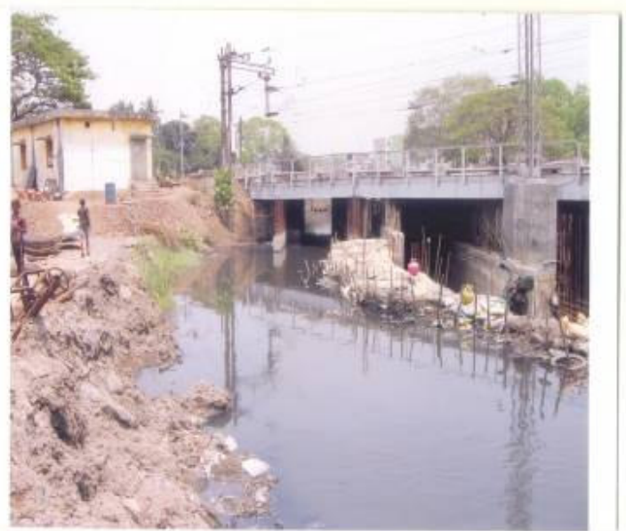
Photograph showing coffer Dam
