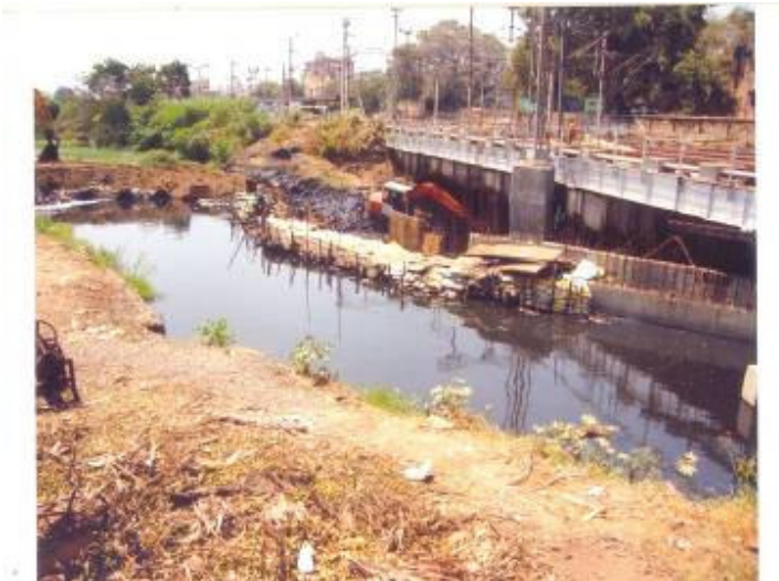
Photograph showing coffer Dam
