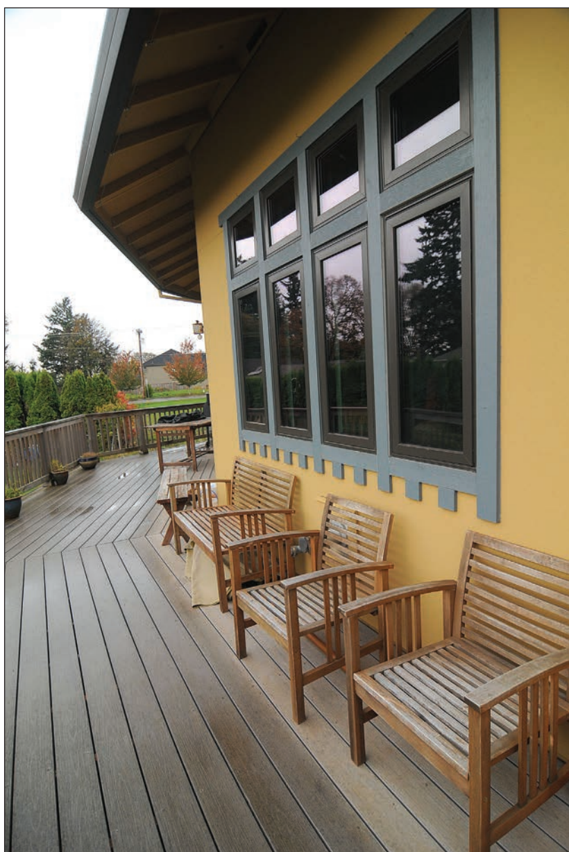
Notice the wide eaves and where the shadow hits on the wall. During summer when the sun is higher in the sky, the eaves protect the house from the heat. In winter, the sun's light and heat will pass through the windows into the home.
