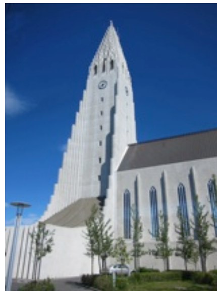
Hallgrímskirkja, designed to resemble lava flowing from a volcano. Photo by Glenn Skoy.
