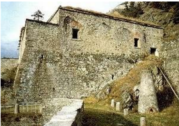
The Powderhouse of Sant'Ignazio with the lightning conductor tower in the foreground
