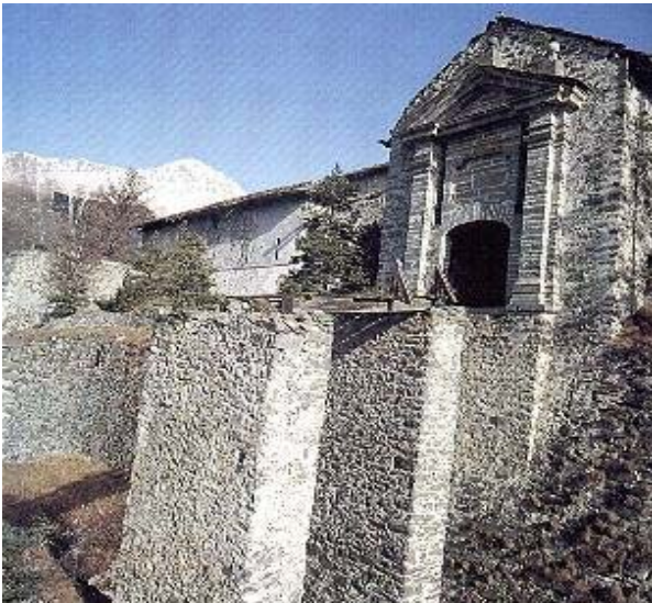
The Main Entrance to the Belvedere Redoubt of the Delle Valli Fort
