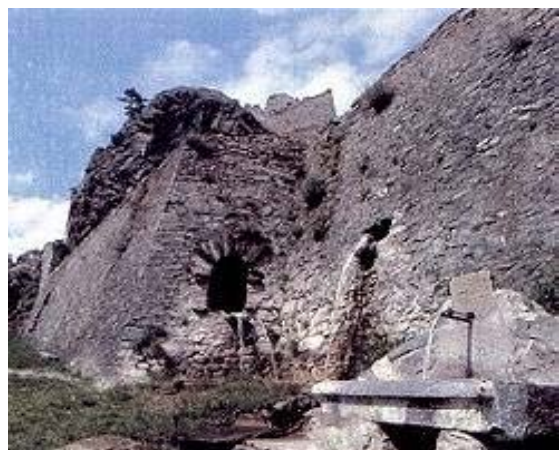
The entrance to the aqueduct at Tre Denti
