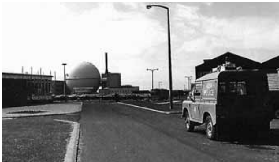
The shut down reprocessing facility at Dounreay in Scotland.
