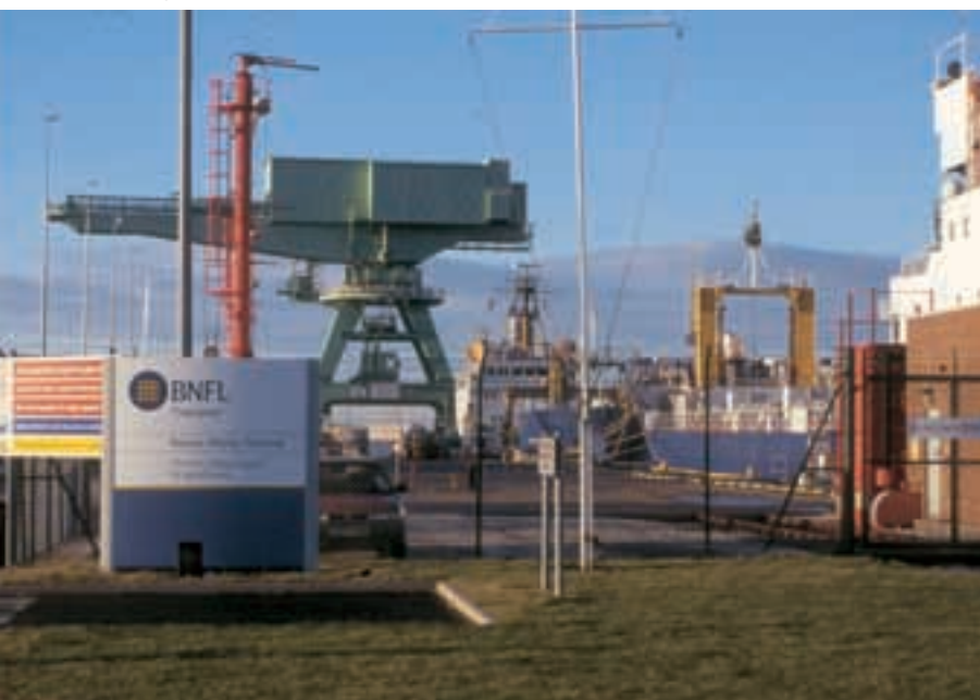
The BNFL quay facility at Barrow
