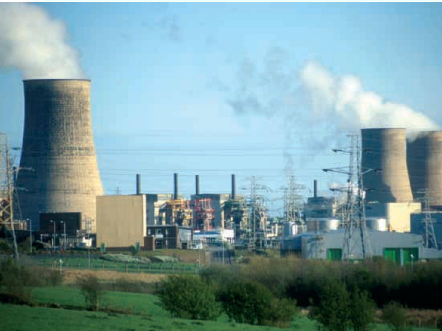
There are four Magnox reactors at the Calder Hall nuclear power plant. This photograph was taken in 1998 when all four reactors still were in operation.
