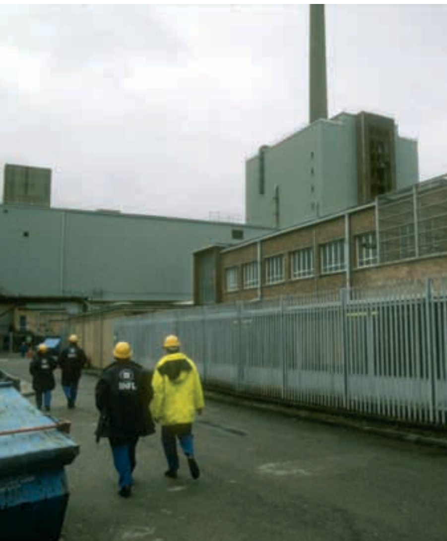
The B204 reprocessing plant.
