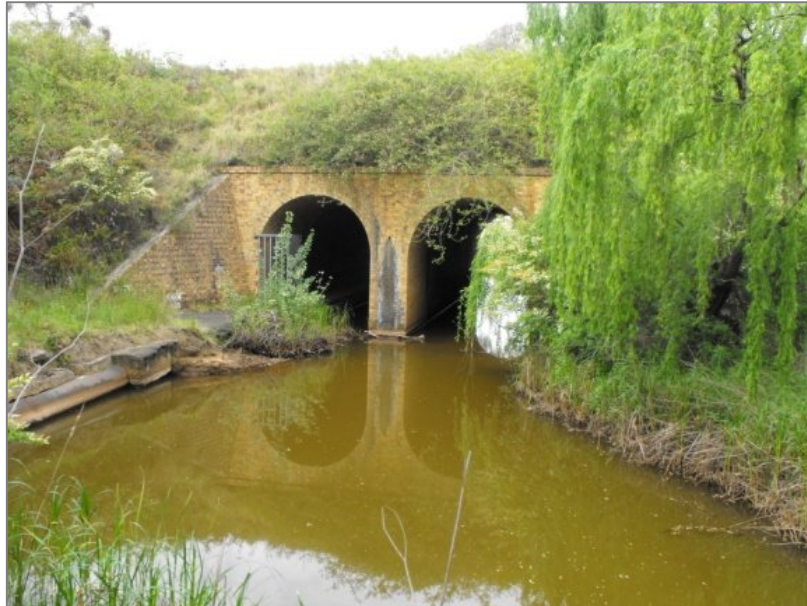
Figure 2.7 Northern elevation of double brick arch culvert over Stony Creek, Farley. Constructed circa 1860. Photograph by Sue Singleton.
