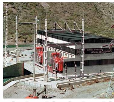
The related power station works consist of the construction of the intake structure, floodgate chamber, the head race tunnel, the surge tank, the penstock, the power station building, the outlet, the 220 kV substation, access roads and an annexed park. Two Francis vertical-axis turbines provide 130 MW generating 400 GWh annual power output (average).
