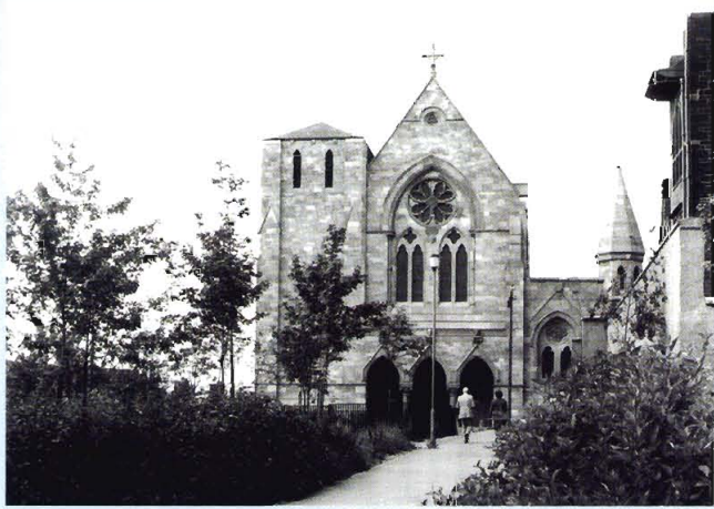
St. Mungo's Church and Monastery
