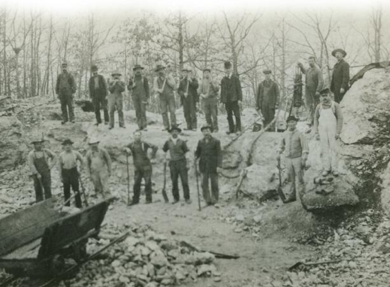
above: Green tourmaline found in the Haddam pegmatite vein. J. W. Peoples Museum, Wesleyan University below: Drilling into a pegmatite in Glastonbury, c. 1890s. The miner (back row, second from right) is holding a "widow maker" drill, so called because the dust could cause a deadly lung disease called silicosis. photo: Charles R. Harte
