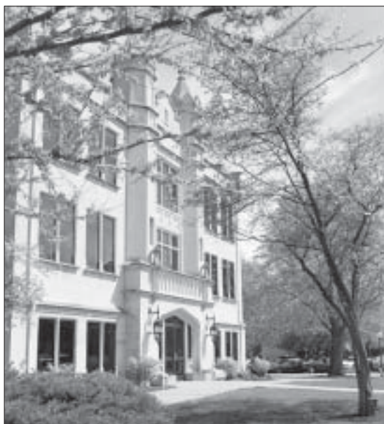
Located in the heart of campus, the Hartmann Center for the Performing Arts originally housed Bradley's first on-campus arena, then known as Hewitt Hall.
