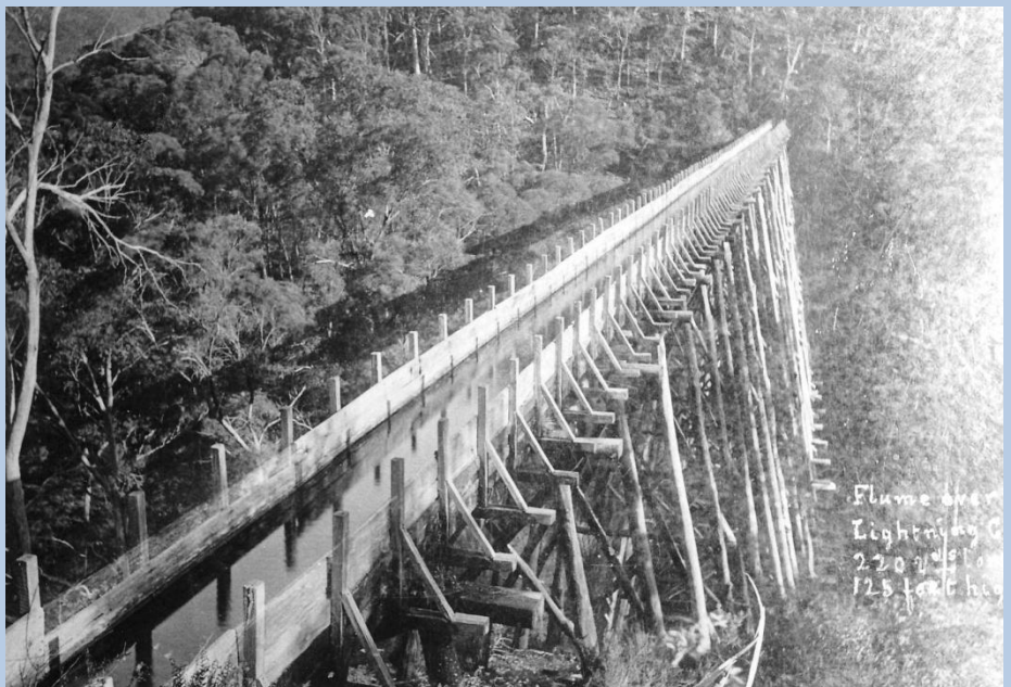
Water flows across the Lightning Flume, wonderfully engineered from timbers cut down at the site. (c1896)
