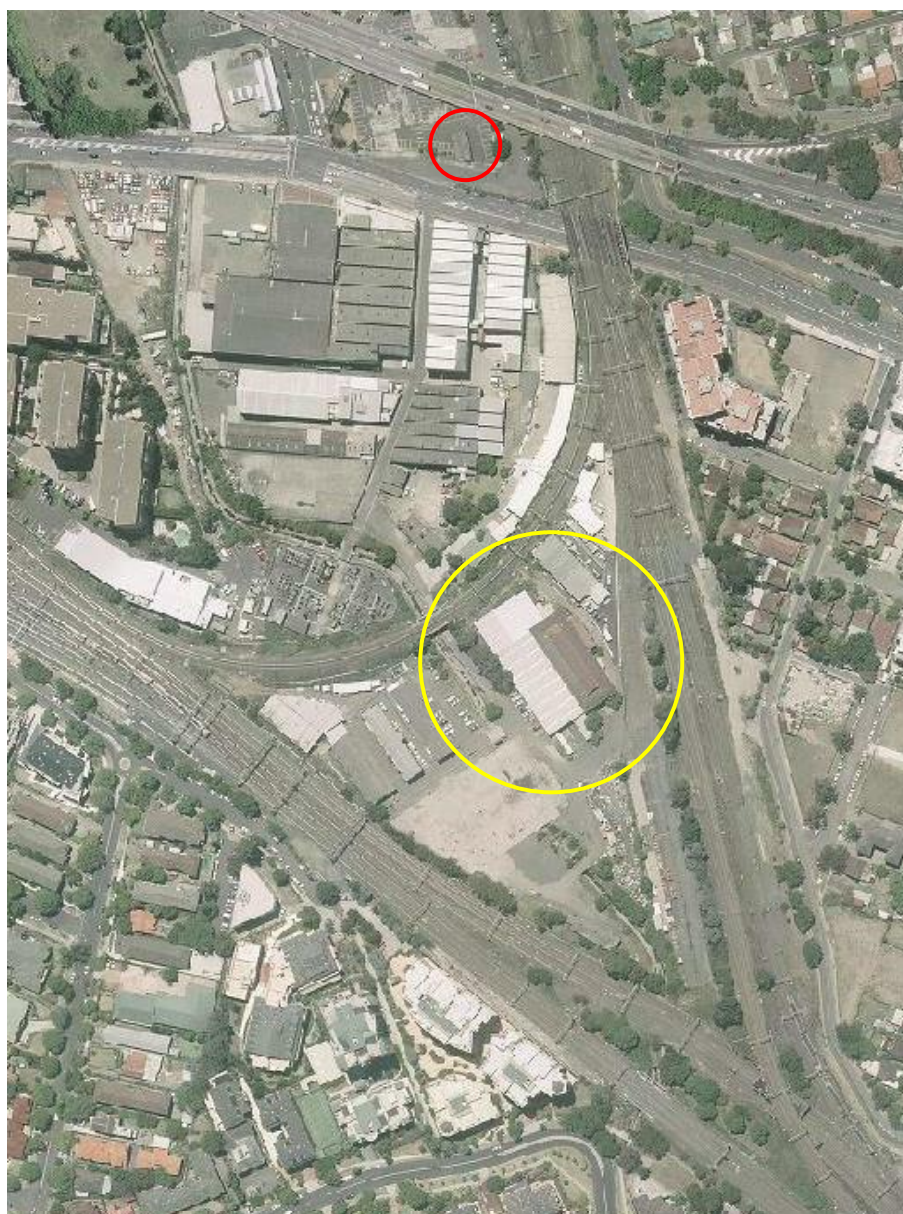
Figure 3.35 Aerial view of the Strathfield Former Substation and Substation 263 in 2008, showing changes in the development of the local environment. The electrical maintenance workshops, which fill the centre of the Strathfield Triangle, have now been demolished. (NSW Land and Property Information; Ausimage © Sinclair Knight Merz)
