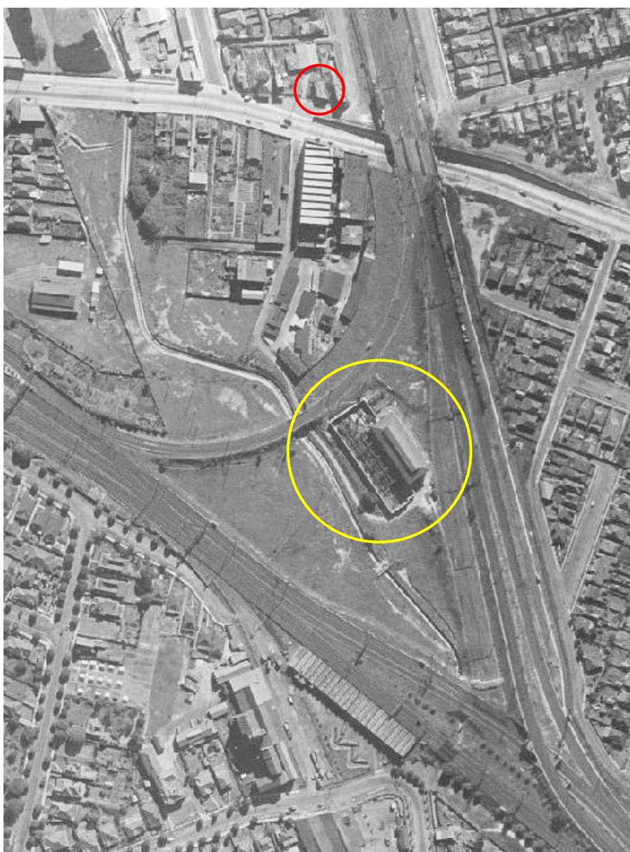
Figure 3.34 Aerial view of the Strathfield Substation (circled in yellow) and Substation 263 (circled in red), 1943. (NSW Land and Property Information; Ausimage © Sinclair Knight Merz 2007 from RTA photography)
