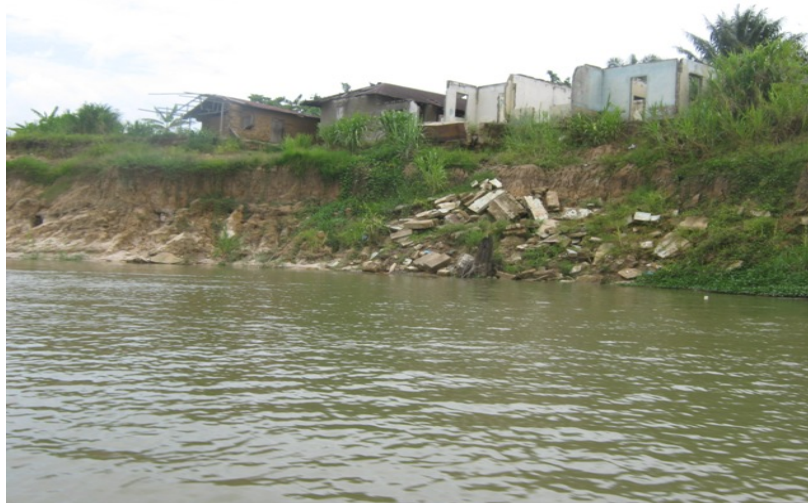
Plate 2. Loss of Physical capital due to river bank collapse in Abari (RULIN field survey, 2010)
