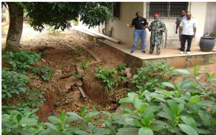
Figure 20 Flood reception pit in Oko, Anambra State
