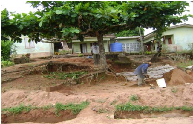
Figure 27 Sand bags are used to fill up eroding areas around homes
