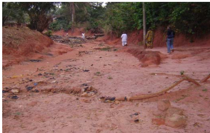
Figure 15 Eroded road at Ngwo-uno in Enugu State
