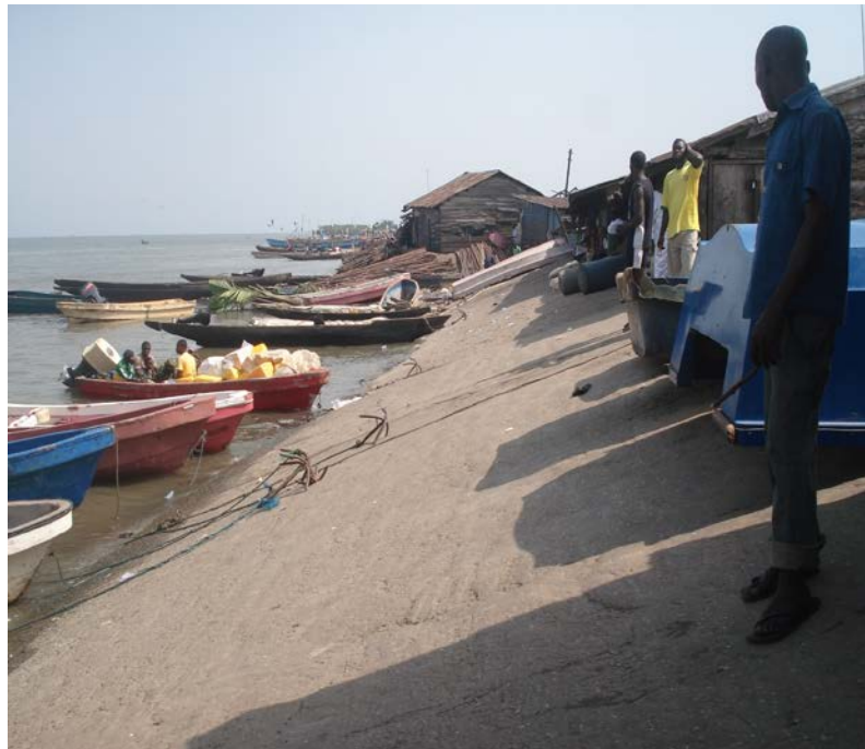
Plate 4: Embankment to check sea level rise at Ibaka beach, Mbo LGA, Akwa Ibom State
