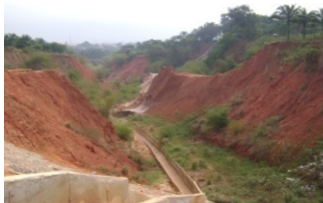
Figure 13 Gully erosion at Ekwulobia in Anambra State
