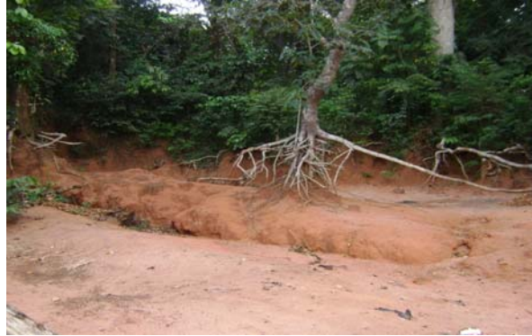
Figure 14 Sheet erosion at Ngwo-uno in Enugu State
