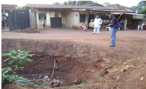
Figure 29 Flood reception pit to check flooding around residential areas in Ngwo-uno, Enugu State
