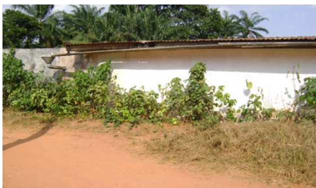
Figure 21 In Oko, Anambra State, water from the roof is not allowed to run off the compound
