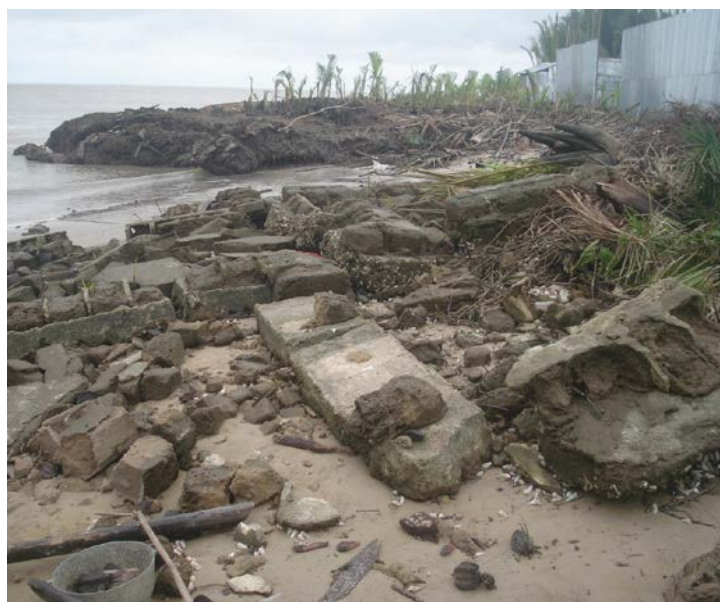
Plate 2: Debris of Brick building destroyed by sea level rise in Ibaka, Mbo, Akwa Ibom State
