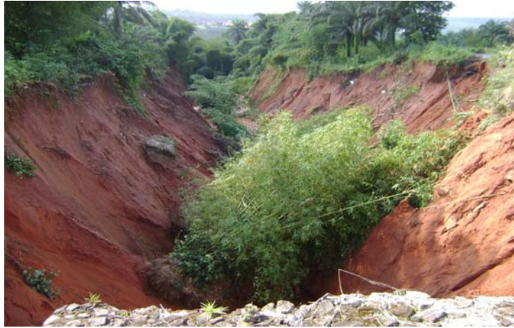
Figure 17 Gully and landslide at Amucha, Imo State
