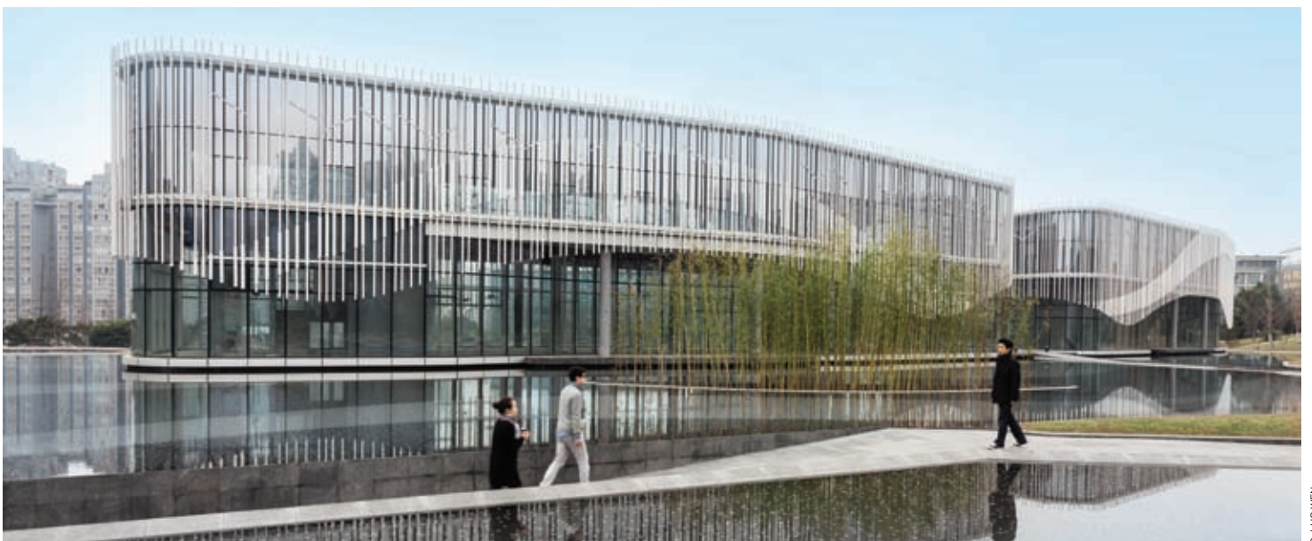
Hassell's Palm Island project is a series of five "floating islands" at the Palm Springs International Garden complex in northern Chongqing, China.
