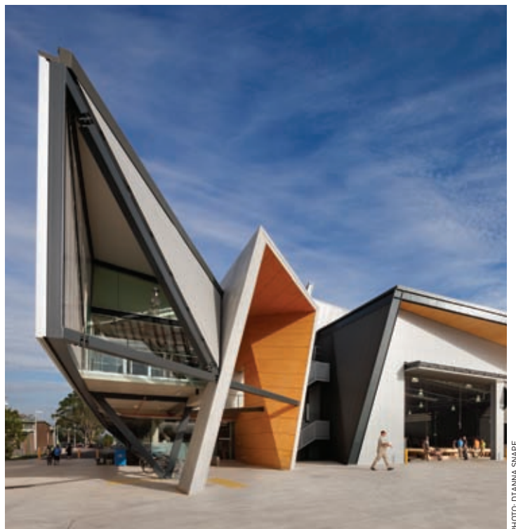
Cox's Sunshine Construction Futures training centre in Melbourne.
