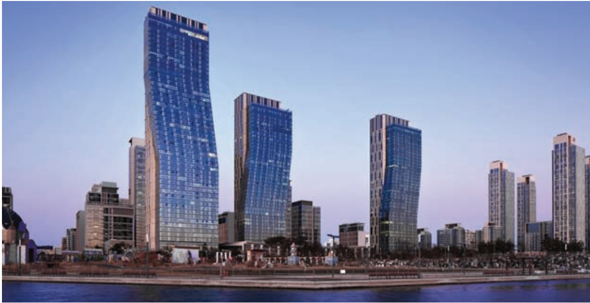
HOK's Central Park I and II mixed-use towers in New Songdo City, South Korea.
