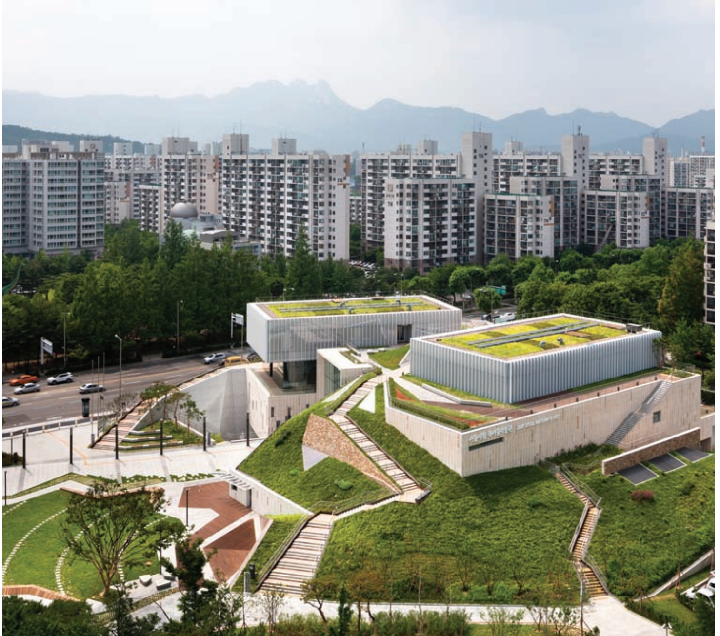
Samoo's Buk Seoul Museum of Art is intended to bring culture and architectural variety to a "monotonous" area of the South Korean capital.
