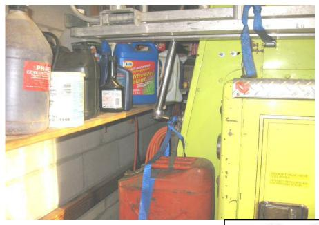
Look carefully at the end of the ladder; it's **touching** the plastic bottle, which is there to protect the back wall of the firehouse. And the grab bar on the fire engine is **touching** the shelf. This total absence of space means the volunteers can't even put their equipment on till the engine is moved out of the building.
