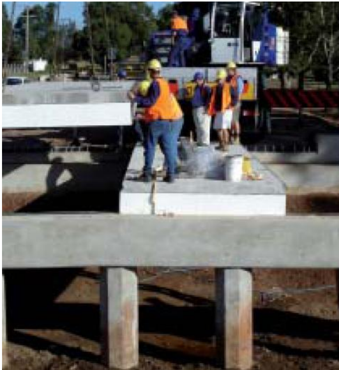
Figure 7: Wagners CFT bridge installation
