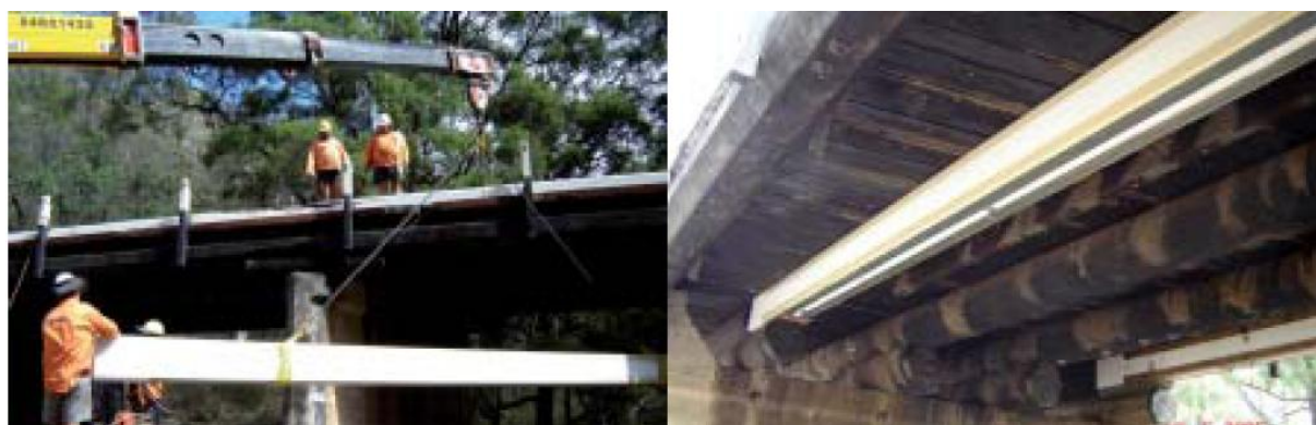
Figure 6: Installation of FCDD girder
