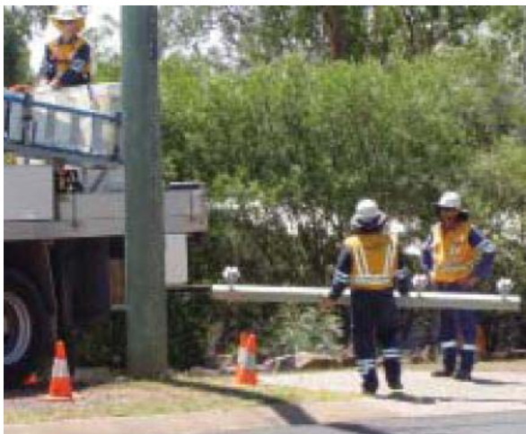
Figure 1: Cross-arm installation
