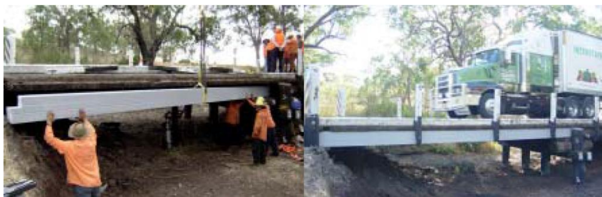
Figure 4: Beam installation and working under load
