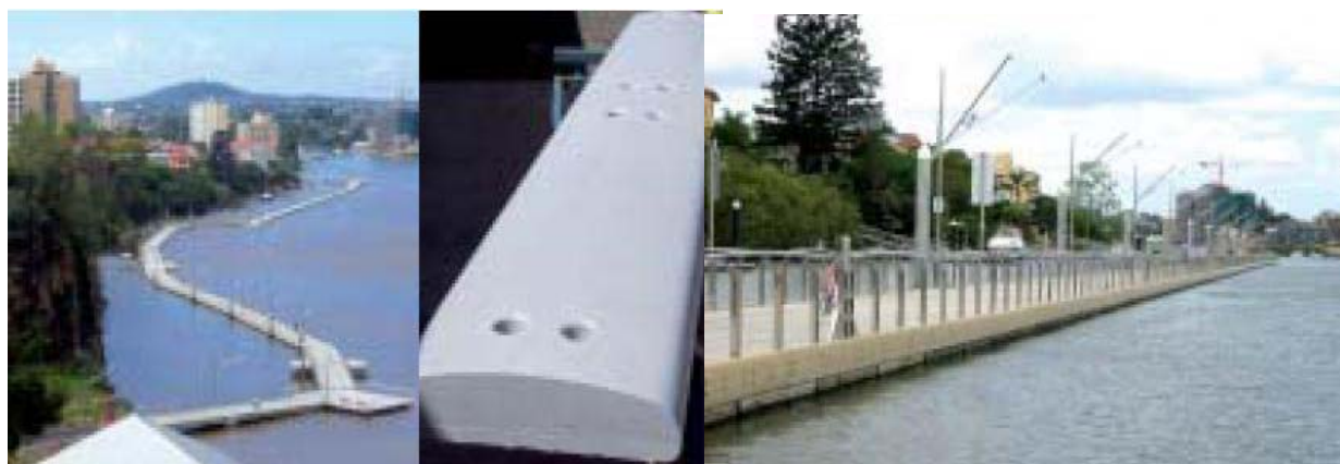
Figure 2: FCDD's fibre composite Waler in the Brisbane City Wharf Project
