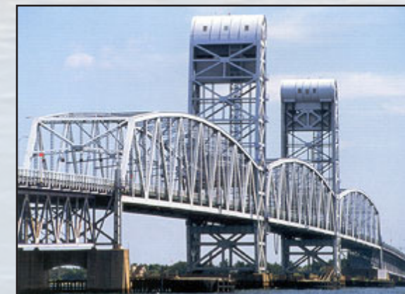
Vertical lift mainspan with through truss flanking spans, Marine Parkway Bridge, New York, NY
