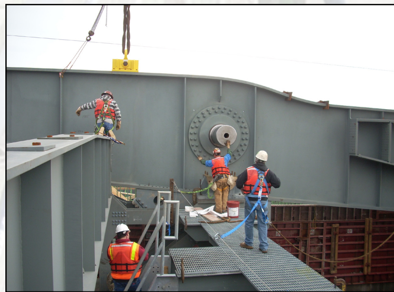
Bascule Girder Erection, Chincoteague Bridge
