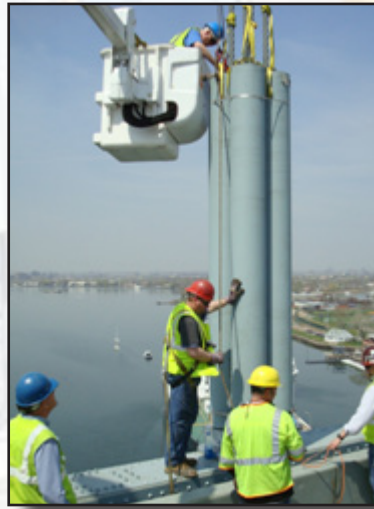
Installing suspender cable protection on Throgs Neck Bridge
