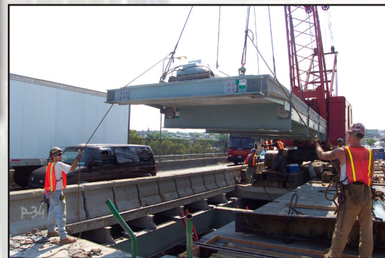
Overhead crane lifting deck section, Triborough Bridge
