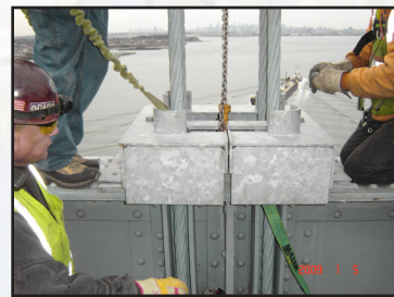
Installing leveling box for suspender protection tubes on Bronx Whitestone Bridge
