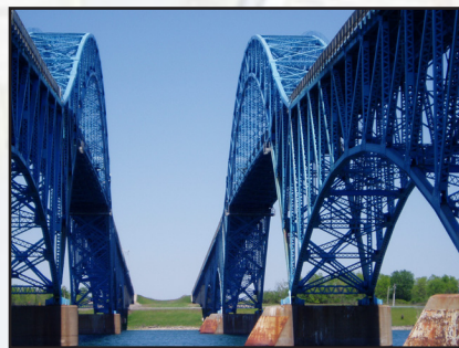
South Grand Island Bridge, Buffalo, NY
