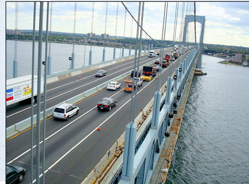
AB is currently working on security improvements for Throgs Neck (above), Bronx Whitestone and Triborough Bridges, in New York City
