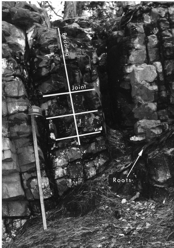
Bald Eagle sandstone near left abutment of Halfway Dam
