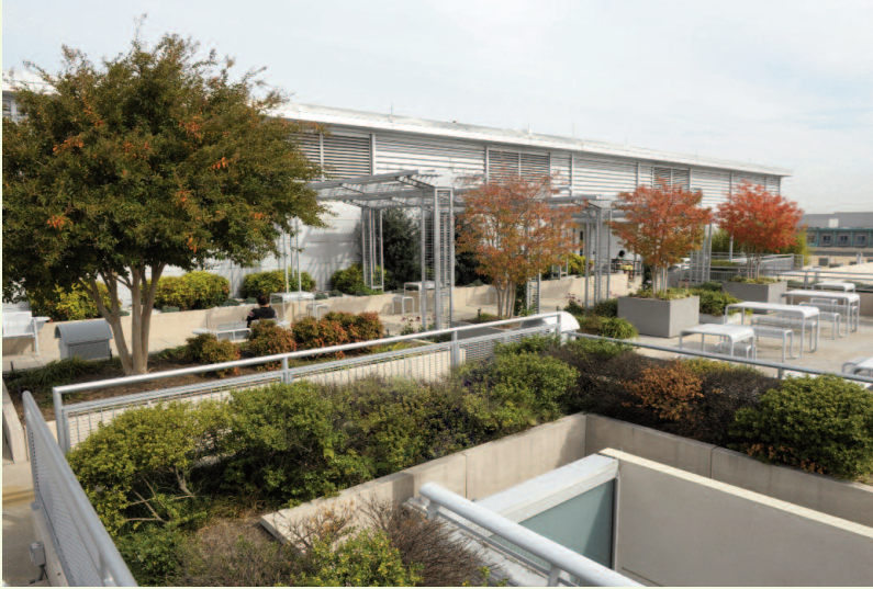
PHI's Edison Place headquarters features a 'green roof' that filters pollutants before runoff joins Washington, D.C.'s water system.
