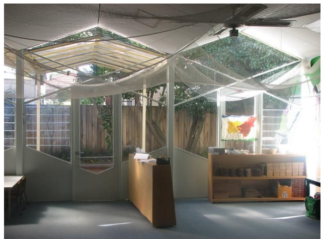
General view of playroom interior, looking north towards porch
