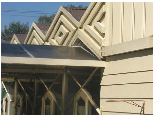
Detail of north facade, showing roof treatment and doors
