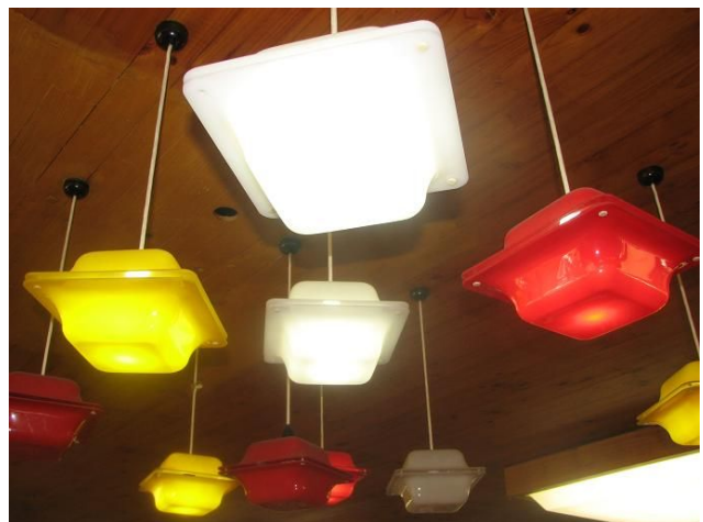
Original light fittings in former children's reading area
