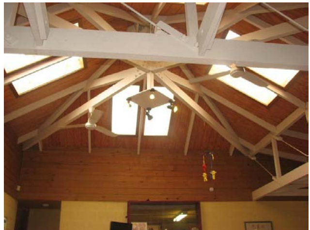
Detail of interior showing exposed roof truss
