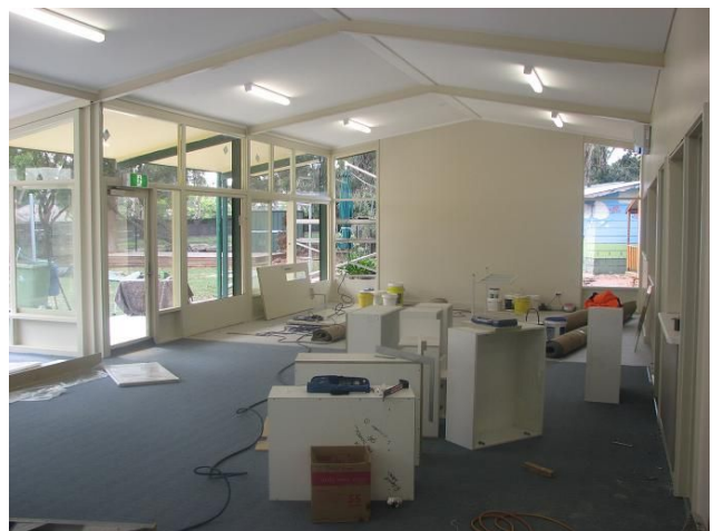
Classroom interior, looking towards rear wall
