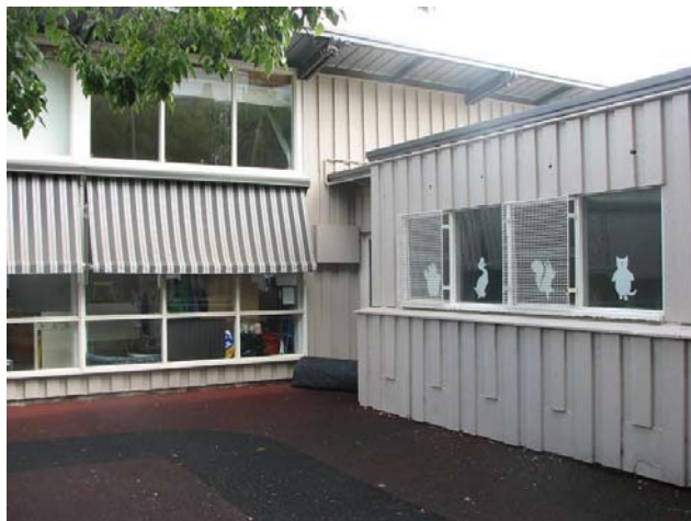
The rear classroom, with service wing (toilets etc) at right
