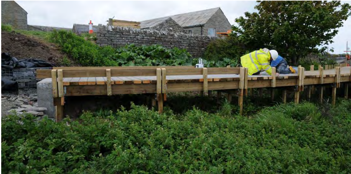
Constructing the boardwalk section of the Brodgar-Stenness footpath
