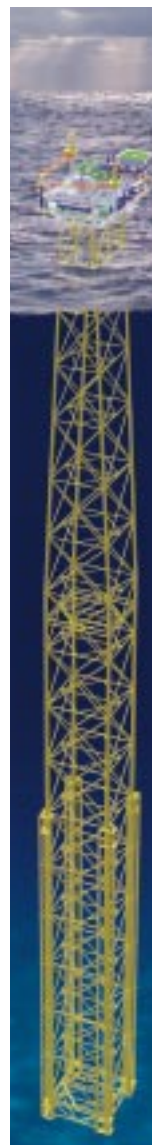
The third generation of the compliant tower for the US Gulf of Mexico (Art by Mustang Engineering).
