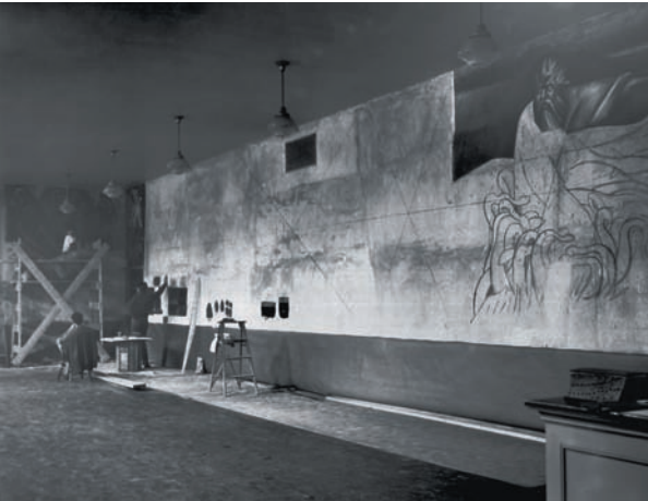
Work in progress on the west and north walls of The Epic of American Civilization (Orozco on scaffold), fall 1932.
