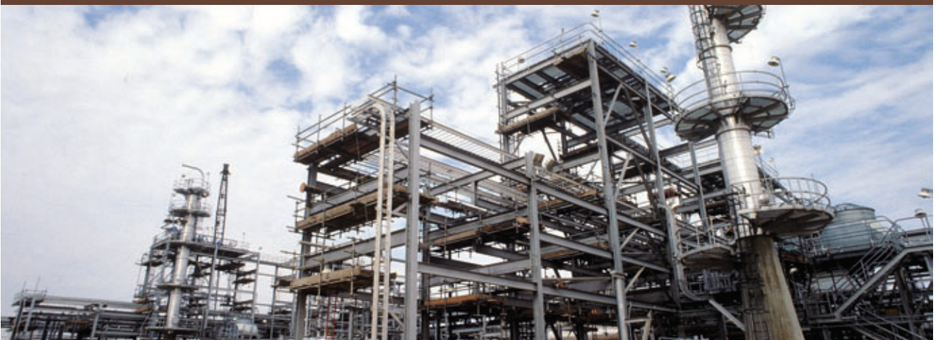
Gas plants such as this one at Haradh are integral to the Kingdom's Master Gas System which processes over 9 billion scfd of gas.
