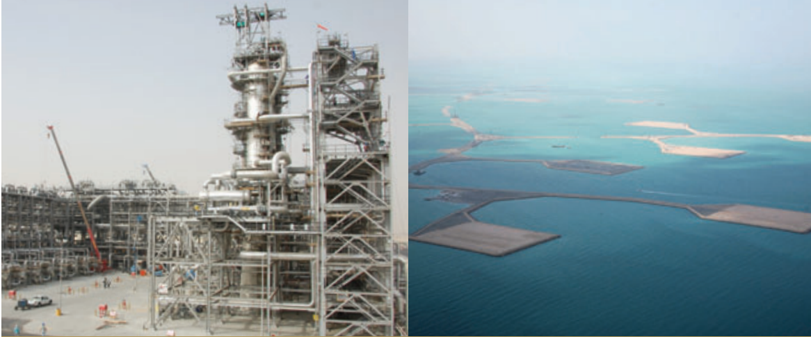
Left: Our 500,000-bpd Khursaniyah crude oil increment started test production in 2008. Right: As part of our Manifa project, we built a causeway and drilling islands in the Gulf.
