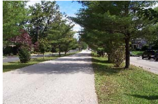
SEPTA Route 103 busway running between East and West Hathaway Lane in Haverford Township
