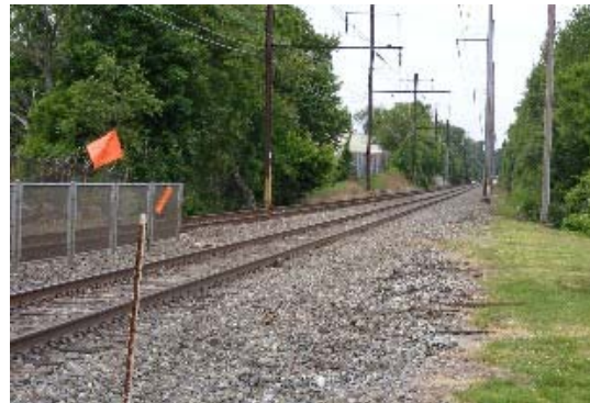
SEPTA Media/Elwyn Regional Rail right-of-way, looking east from the Clifton-Aldan station in Aldan Borough
