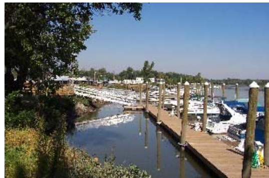
An example of a facility that can support a water trail – Ridley Township Municipal Marina on Darby Creek
