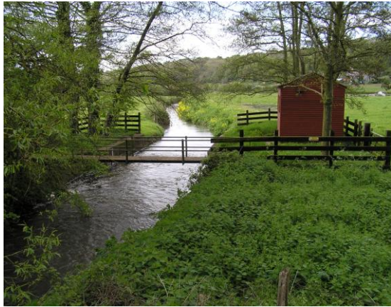
Environment Agency remote monitoring station on the Land Yeo at Wraxall House ST483715
