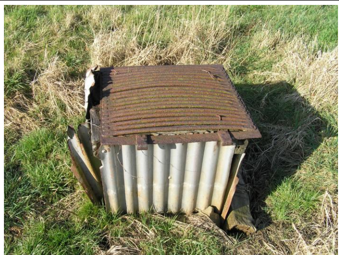
Access shaft for Jacklands Tunnel at Moored Spout (26 February 2012) ST 4669 7155
