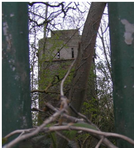
Engine house at Middle Engine Pit. The tank on top of the tower was used to store water for the Elms private house. ST 482 706
