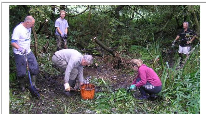
Clearing one of the ponds in the carr at Moorend Spout. (A carr is a wet woodland, usually with willow and alder). This pond is more like a swamp and it can be dangerous! ST 4661 7154
