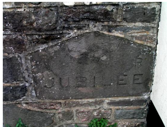
Stone engraved with 'Jubilee' now built into a wall at the Friendship Inn. This was at the top of the water tower.
