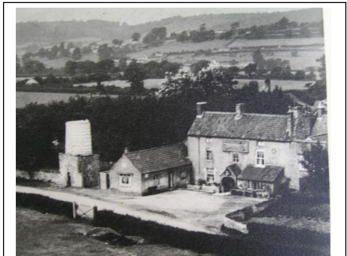
Water pumped from the Land Yeo was stored in a reservoir adjacent to the Friendship Inn, (white tower to the left)
