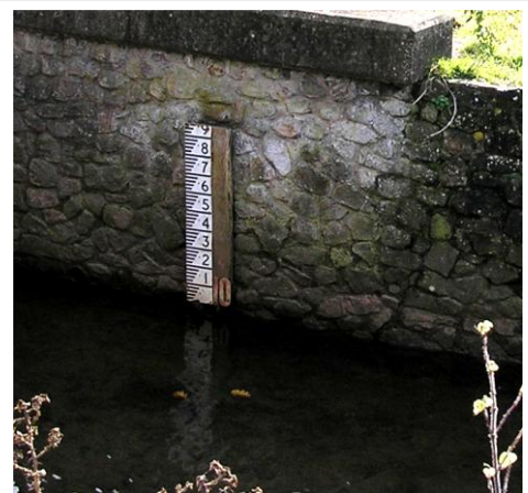
Gauge at Jacklands Bridge marked at 10 cm intervals ST 469 717
