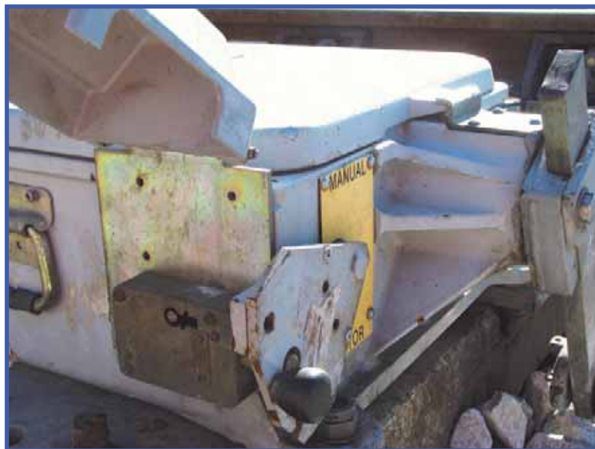
Plungers are provided for the local release of the points locking in the event of track circuit failure.
