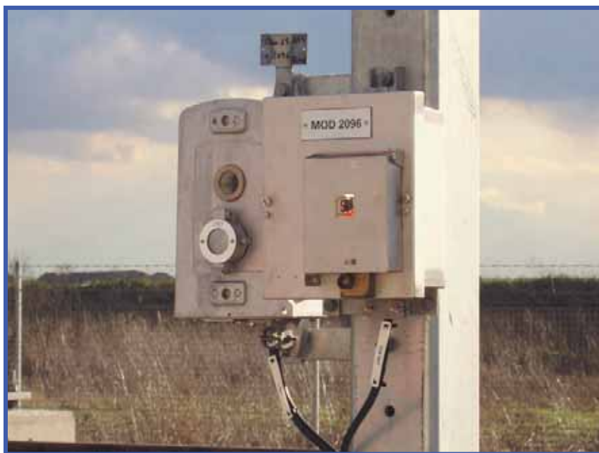
Plungers are provided for the local release of the points locking in the event of track circuit failure.
