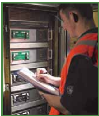
The SSI interlockings for Coruche, near Lisbon are being replaced by the latest WESTLOCK units.
