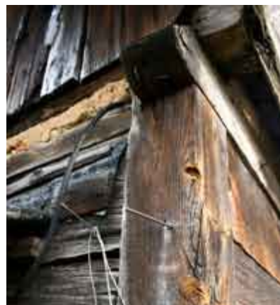
Post and board construction in Zamęty
