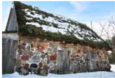
Cowshed from split stones originating from fields nearby, in Piskory
