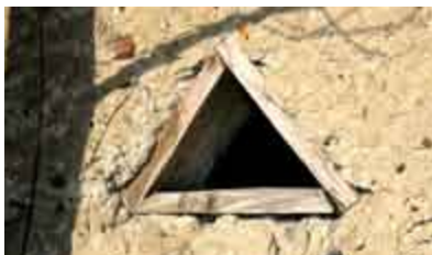
Small window in a farm building in Zapowiednia
