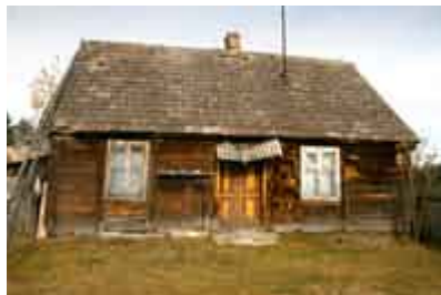
Tiled roof in Zamęty
