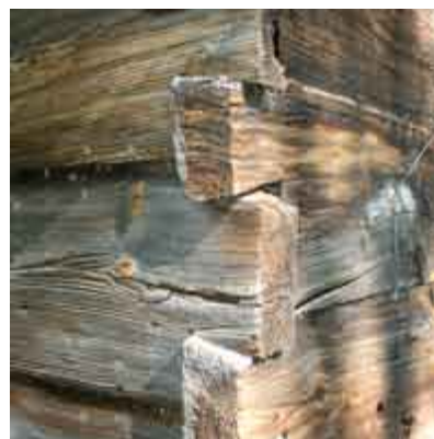
Saddle notch construction in Borowiec Nowy
