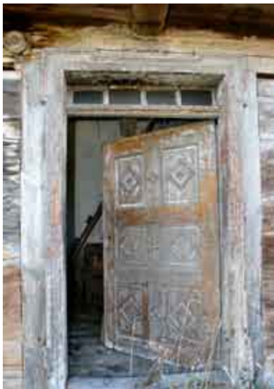
Charming abandoned homestead in Wierzchy
