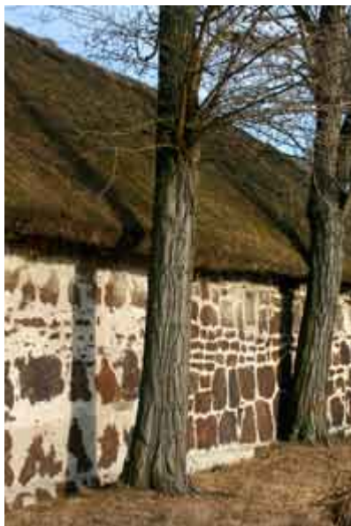
Patched wall from bog iron in Czarny Bród
