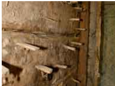
Stakes driven into boards for supporting clay plaster in Wierzchy
