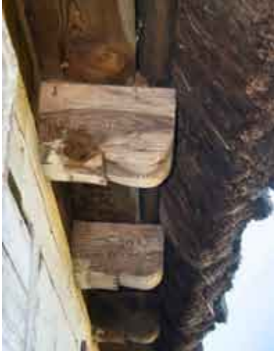
Extended joists for fixing roof in Wierzchy
