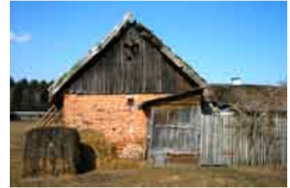
Cowshed and outhouse in Kolonia Obory
