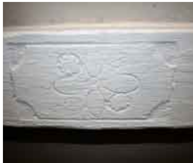
House joist in Stara Kaźmierka
