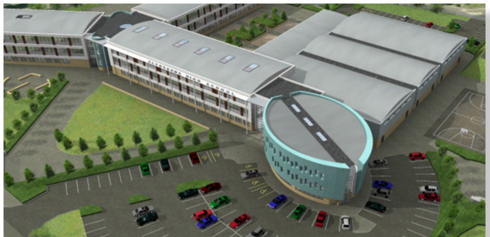
Park Mains High School, Erskine
