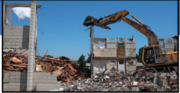
Demolition crews leveled the former residential complex over the summer.
