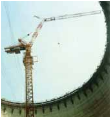
Liebherr 180 HC-K articulated saddle jib climbing crane on its first job; construction of the 150 m high cooling tower in Gösgen, Switzerland in 1976. Note the horizontal rope anchoring system that had to be used at three levels
