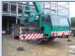
50 t Liebherr LTM 1050-1, 1997
