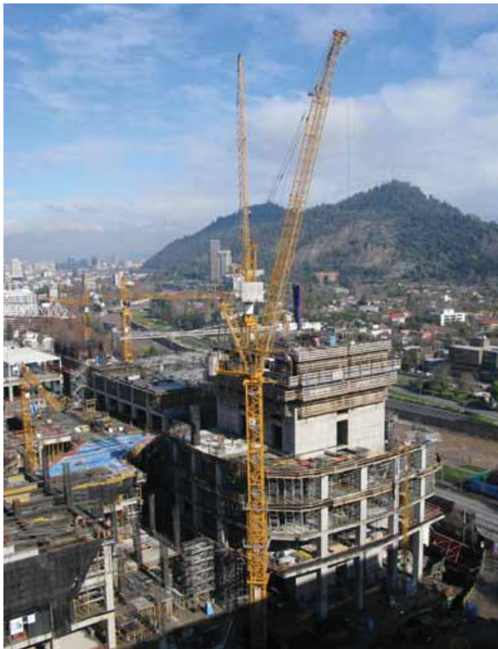
Liebherr top-slewing luffing jib tower cranes work on the 694,000 square metre Costanera Center in Santiago, Chile
