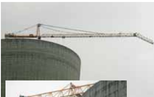
Real jib shortening started with the folding of the jib head section after removal of the top chord connecting bolt
