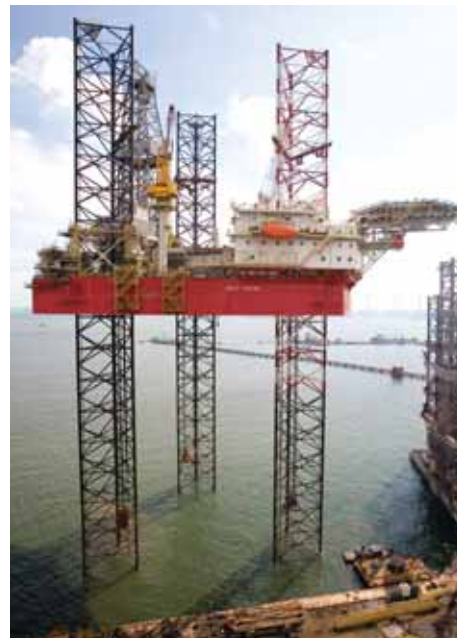
◆ West Triton, the 6th BMC Pacific 375 jack-up rig delivered by PPL Shipyard
