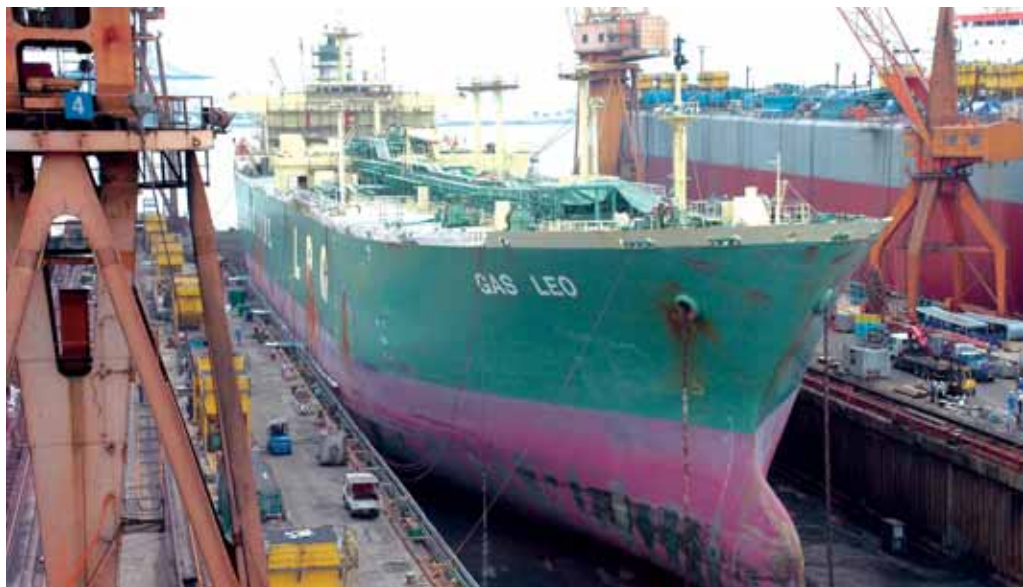
◆ Gas Leo undergoing repair and maintenance works
