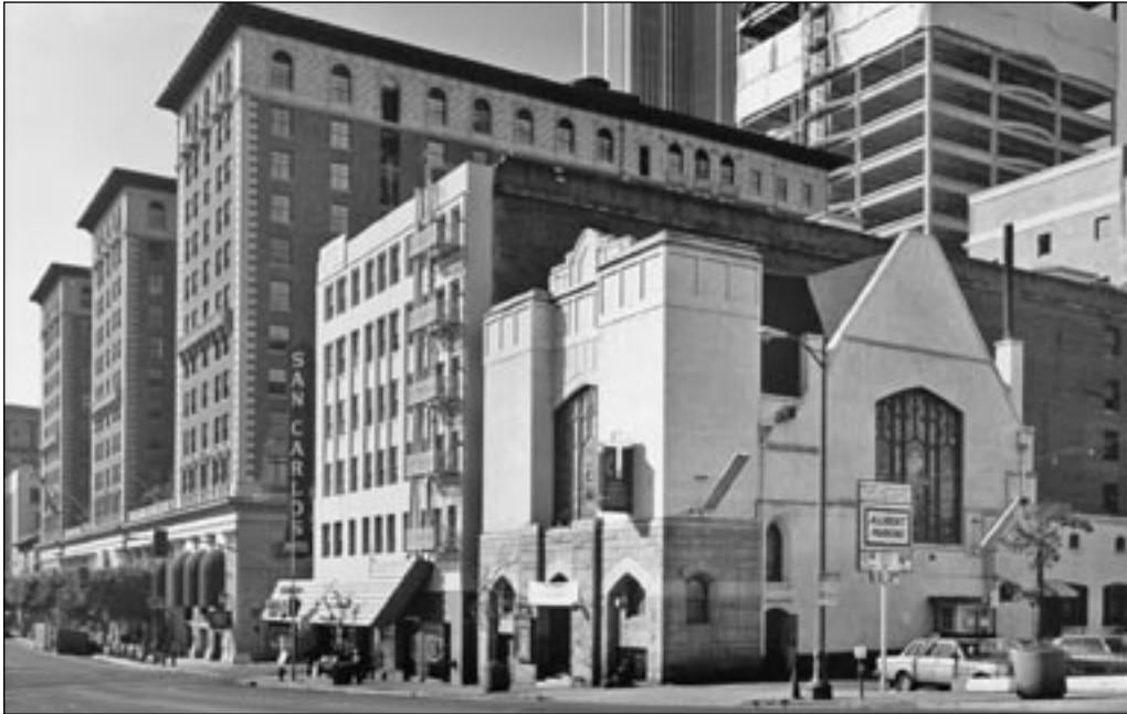
The Biltmore tower is pictured under construction in 1985. The renovation included the opening of the Grand Avenue lobby, formerly the music room and later the location of the headquarters for the 1960 Democratic National Convention. In the forefront are the First German United Methodist Church (opened in 1910) and the San Carlos Hotel, built about 1920 and housing the second Googie's Coffee Shop. Both were demolished in 1988 for the Gas Company Tower. (CHS.)
