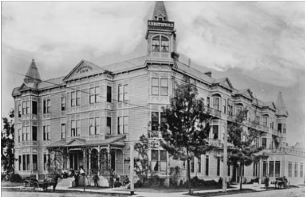
The building pictured about 1890 was located on the southwest corner of Hope and Eighth Streets. D. W. Hanna constructed the building in 1887 for Los Angeles College, a boarding school for girls. It was bought in the 1890s by Abbot Kinney and operated as Abbotsford Inn and had 100 rooms. First Methodist Church purchased it in 1914 and demolished it in 1921 to build a new church building. (CHS.)
