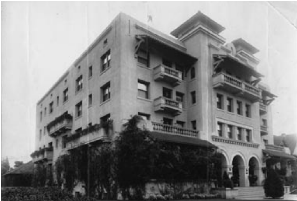
George W. Kitchen built the Shoreham Hotel, located at 666 Carondelet Street south of Wilshire, in 1911. Its four-story Mission-style structure held 100 rooms and was styled as a residence or family hotel. (CHS.)
