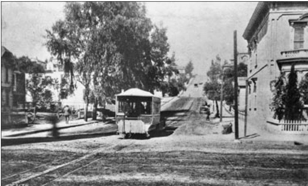
The Second Street Cable was the earliest access line over Bunker Hill. In operation from 1885 to 1889, it ran from Spring Street to its western terminus at Belmont Avenue on Crown Hill. Andrew Hallidie constructed the line. He was the builder of San Francisco's famed cable line. This 1889 view shows a car making its way down Second Street at Broadway. (CHS.)
