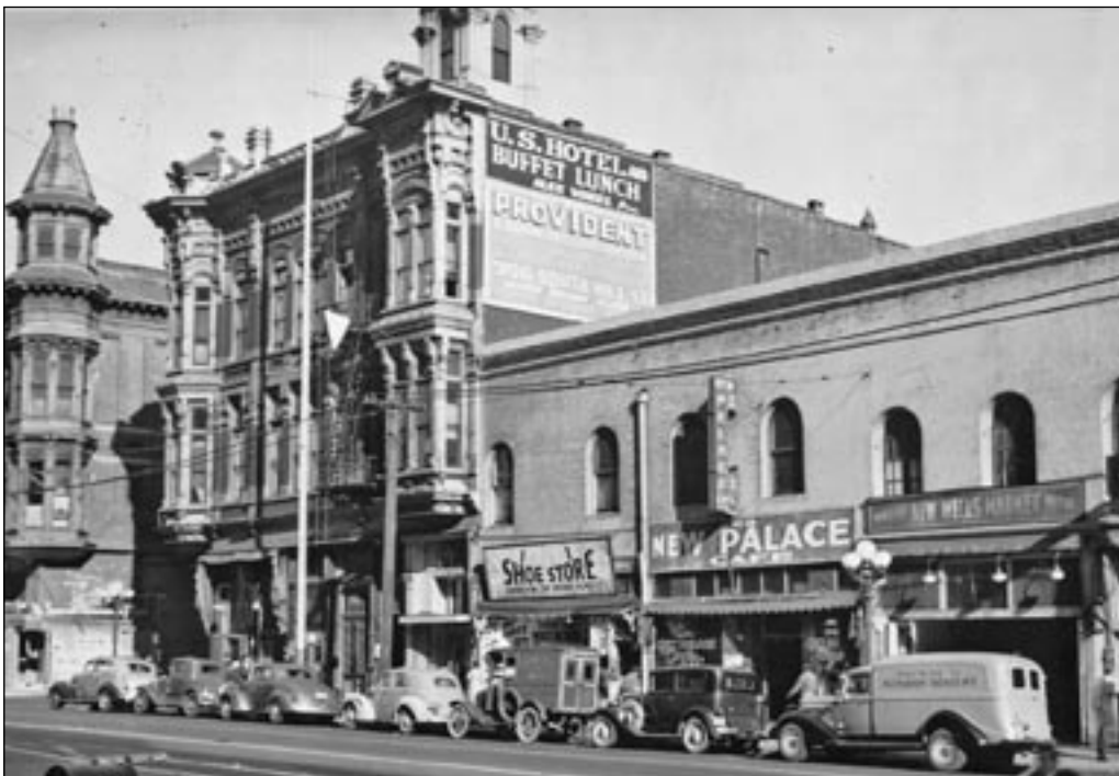
The U.S. Hotel was built around 1863 at 170 North Main by Louis Mesmer, then remodeled and expanded in 1886. The hotel attracted a swanky crowd and served the “best two-bit meal in Southern California” in its dining room, according to advertisements and articles published in the Los Angeles Times . By the early 1930s, it was still owned by the Mesmer family and lodged only men, many on public assistance. (CHS.)
