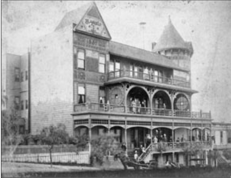
The St. Angelo hotel at 237 North Grand Avenue was built during the boom of the 1880s when it was advertised as a European family-and-tourist rooming house. During the next few decades, the hotel and its guests were mentioned in the society pages. (CHS.)
