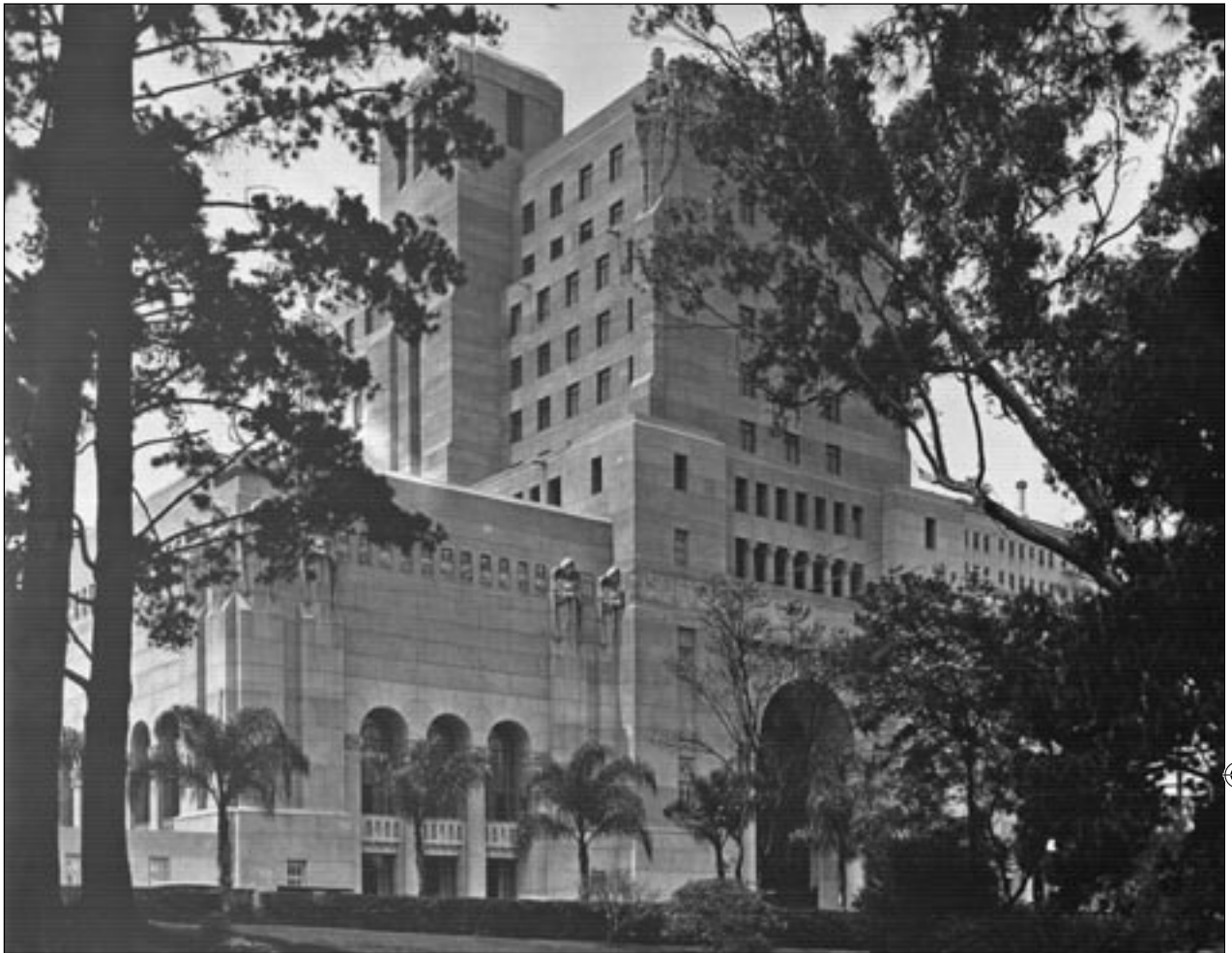
The Lodge 99 of the Order of Elks Building, located at 607 South Park View Street, was designed by Curlett and Beelman and built in 1925 and 1926. It was sold in 1966 and renamed Park Plaza Hotel. Seen here in 1930, the Beaux-Arts, etched-concrete structure is half mastaba, or squared-off Egyptian pyramid, and half nine-story hotel with 160 rooms that rise out of the mastaba. A pair of crystalline plinths rises to become molded architectural warrior angels at each face of every corner, which are topped by a squashed urn. The hotel also has angels that are about twice as high as the others, guarding plinths along each side. The brilliant Art Deco interior of the hotel is a popular site for filming, weddings, and parties. The Art Deco design is apparent in the oversized stairway, the murals by Anthony Heinsbergen, the vaulted ceilings in the lobby, and the three ballroom-type halls. (Examiner.)
