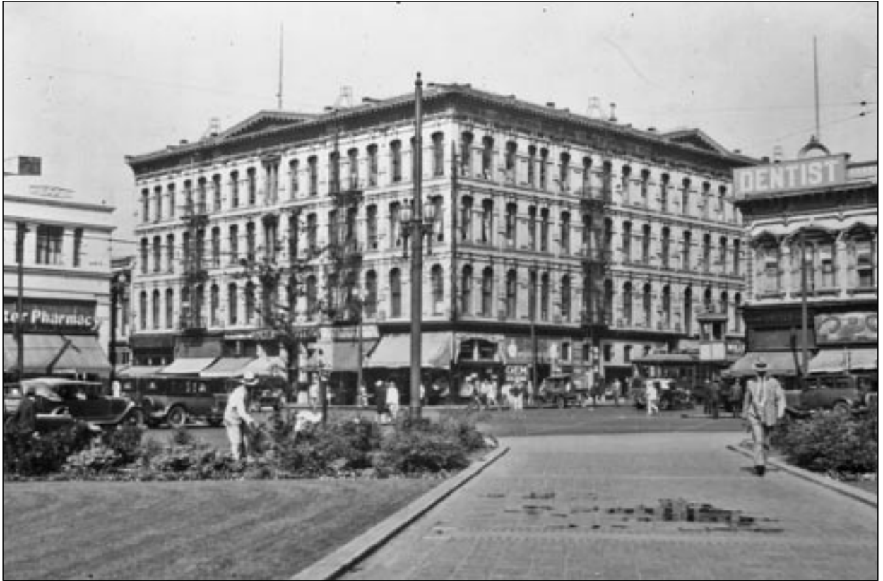
Remi Nadeau bought the plot on the southwest corner of First and Spring Streets in 1872 for $20,000. He opened Hotel Nadeau in 1882 with a grand ball attended by Southland's elite. The hotel installed the first electric elevator in Los Angeles. In this 1931 photograph, the Nadeau is seen across the lawn of Los Angeles City Hall, which was constructed in 1921. The hotel was demolished shortly after this picture was taken and replaced by the Los Angeles Times Building, which was designed in 1935 by Gordon B. Kaufmann in the Monumental Moderne style. (CHS.)
