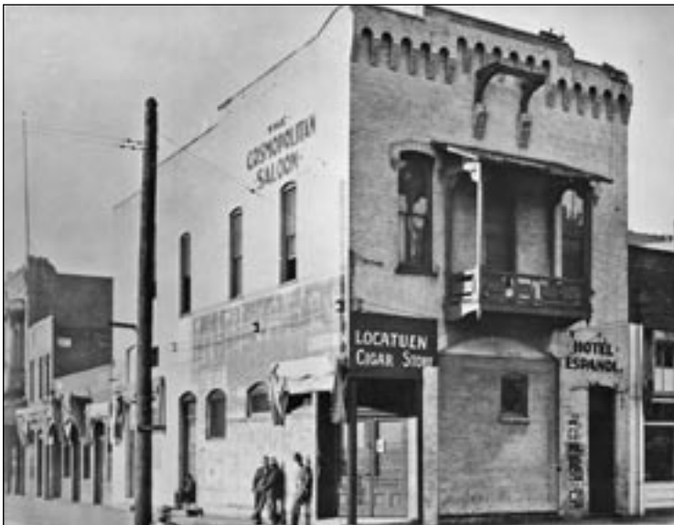
The Old Fire House at 126 Plaza Street was designed by W. A. Boring in 1884. It was the second firehouse built by the city. Today it is the oldest standing firehouse in Los Angeles. In this c. 1920 photograph, Hotel Español occupied the second story, and the Cosmopolitan Saloon and the Locatuen Cigar Store were located below. (CHS.)
