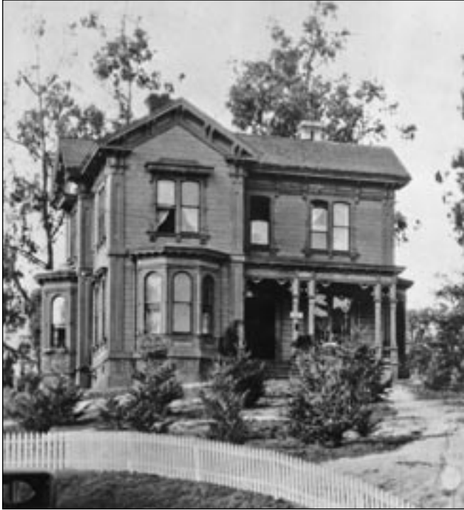
Pictured here c. 1918 is the Foy residence, which stood on the northwest corner of Figueroa and Seventh Streets and later became the location of the Statler Hotel. In the 1920s, the Foy residence displaced the Arnold building, which housed the Hudson and Essex motorcars. By the 1930s, Paul G. Hoffman Co. Inc. Studebaker car dealership stood north of the building. (CHS.)
