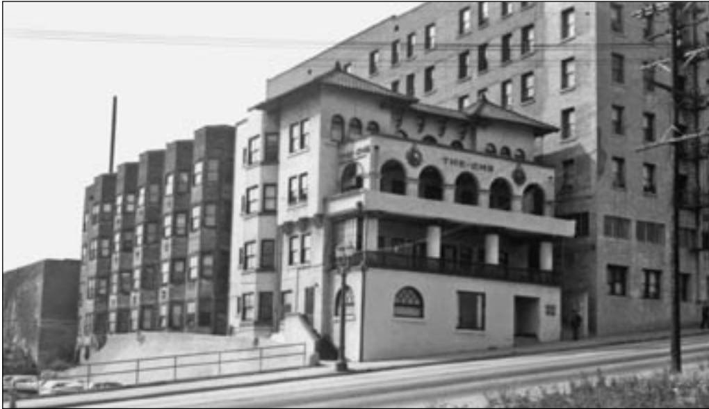
The 40-unit Ems Hotel at 321 South Olive Street near the top of Angels Flight railway was built around 1905 by contractor W. H. Griswold for the owner, Charles C. Emswiler. The image reveals the Mission-style architecture is a facade. Behind its front, is the continuation of a plain frame building. The California Plaza complex has replaced the Ems. (Community Redevelopment Agency of the City of Los Angeles.)
