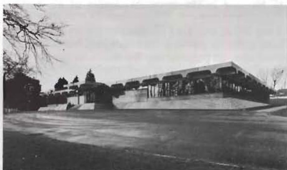
Offices for Conder Kingsworthy Court, Winchester Architect: Sydney Kaye, Firmin and Partners Contractor: Tarmac Construction Ltd.
