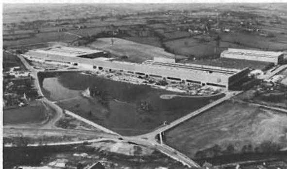
Production, Research and Service Complex for J. C. Bamford Ltd., Rotherham Architectural Services: Staff Architect's Department, J. C. Bamford Ltd. Contractor: R. M. Douglas Ltd.
