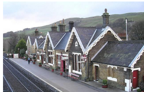
Settle Station (© John Illingworth). Arq. de la Estación: John Holloway Sanders (1825-1884), http://www.victorianweb.org/technology/railways/81.html
