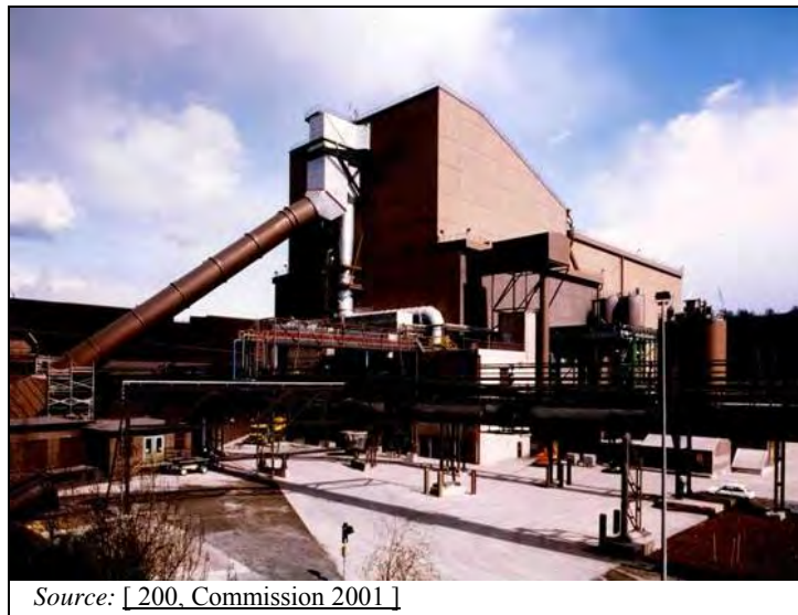
Figure 8.1: Electric arc furnace plant
