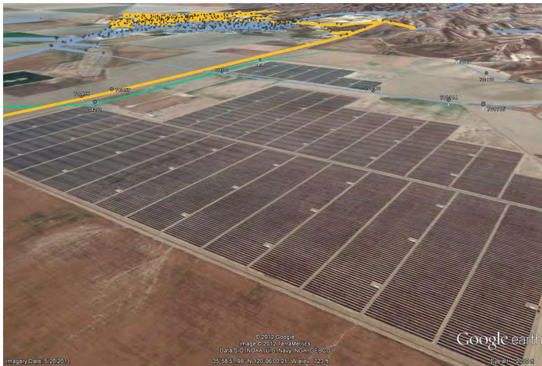
Figure 4: Aleatico Park Photovoltaic Project
